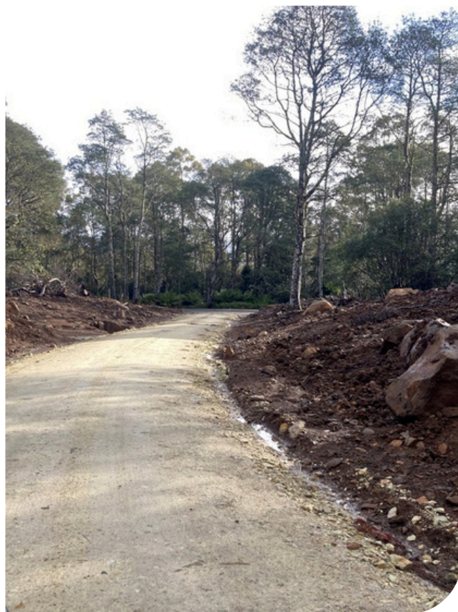
The new entrance constructed by STT to the project site area, off Cradle Mountain Road.
