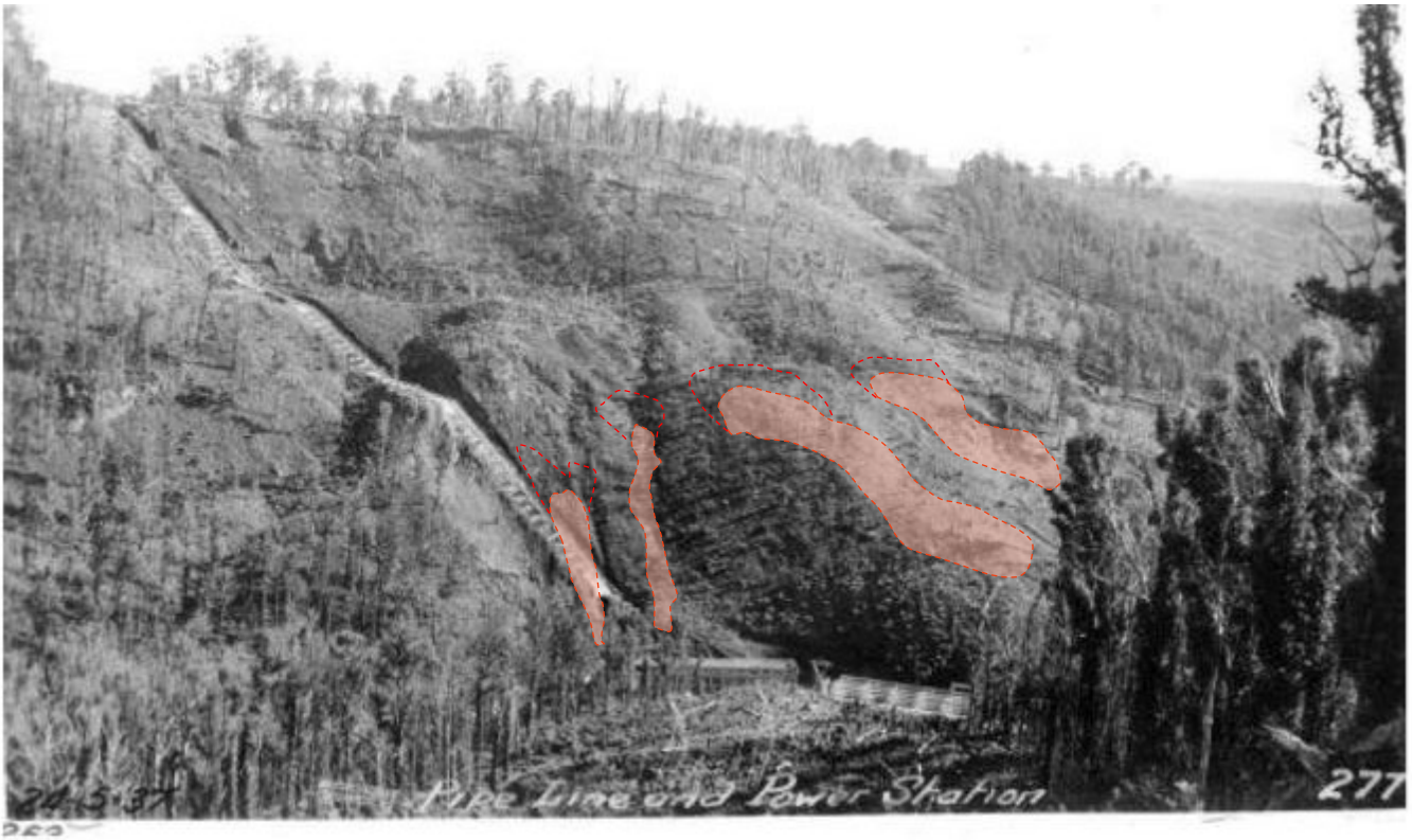
Photo 3: Oblique view of the wider Tarraleah slope during penstock construction in 1937. Note the lack of mature vegetation on the slope. Localised shallow debris slide highlighted in red and provide context for slope evolution and detachment timing.
