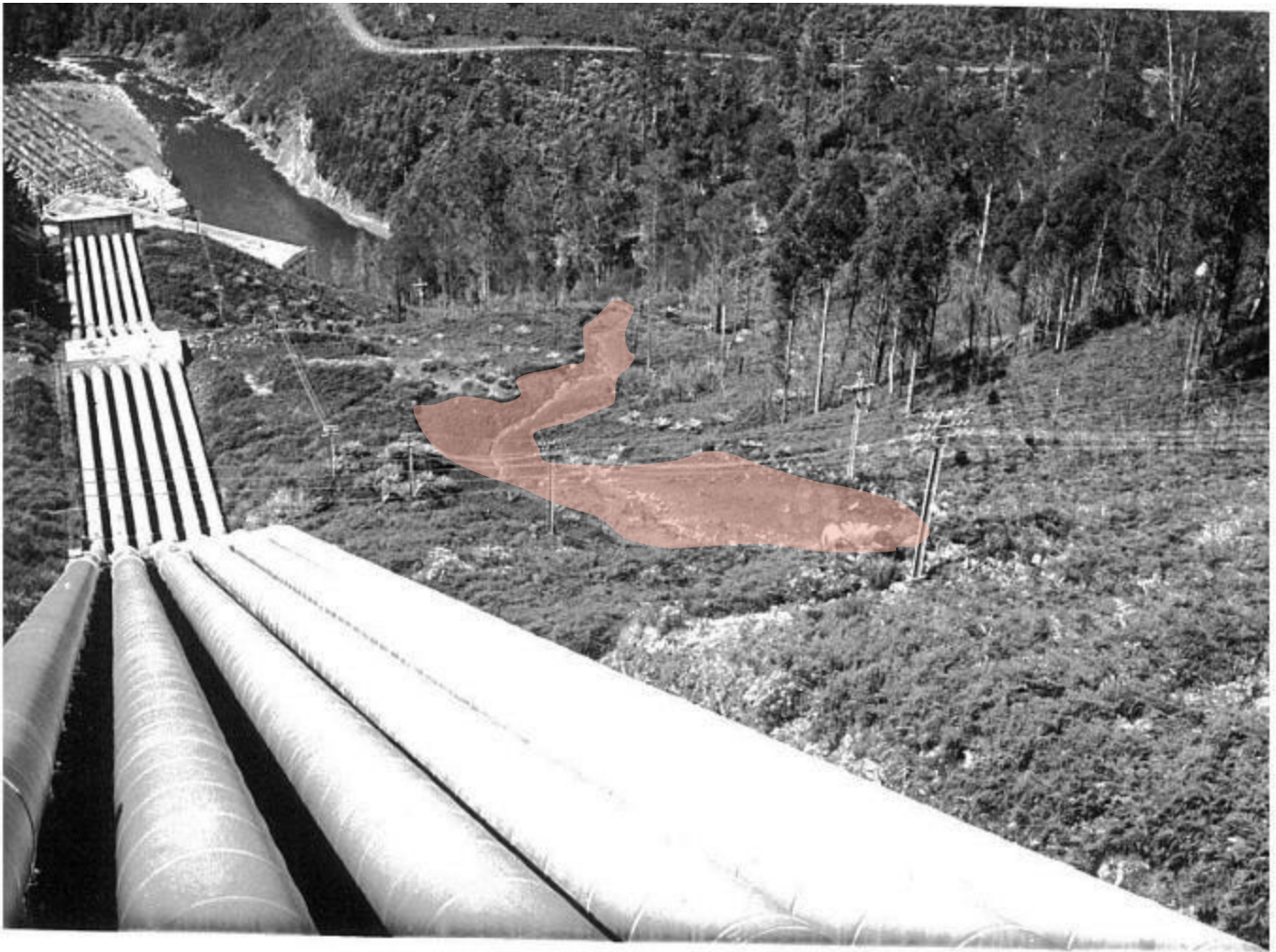
Photo 2: View looking down penstock alignment following release of a localised mudslide/debris flow on the downslope side of the penstocks in 1971 (highlighted red). Photo source: Geologist_Landslip at Tarraleah Penstock_17 Jan 1972.pdf.
