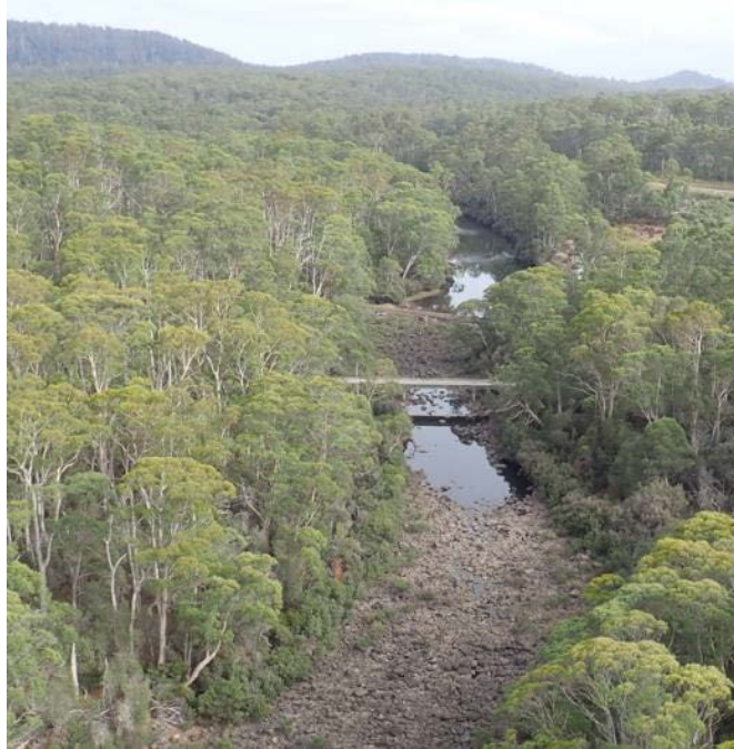
Figure 6.16: Derwent Pumps Weir (upstream of bridge) restricts flow, enabling water to be pumped from the river. Flow direction is from top to bottom of photo (Photo 6 in Figure 6.11).
