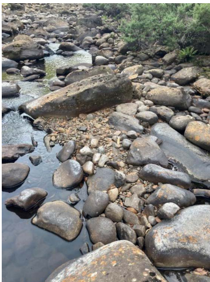
Figure 8.9: Patches of mobile substrate typically comprise gravels, pebbles and cobbles in the lee of large boulders in the River Derwent downstream from Clark Dam.
