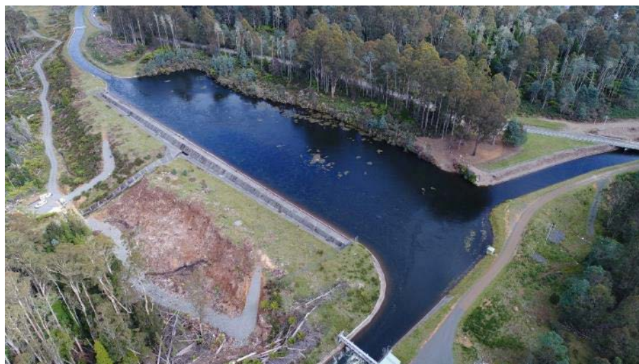
Figure 6.65: No. 1 Pond, No. 1 Canal enters from top left and discharge from No. 2 Pond enters from top right.
