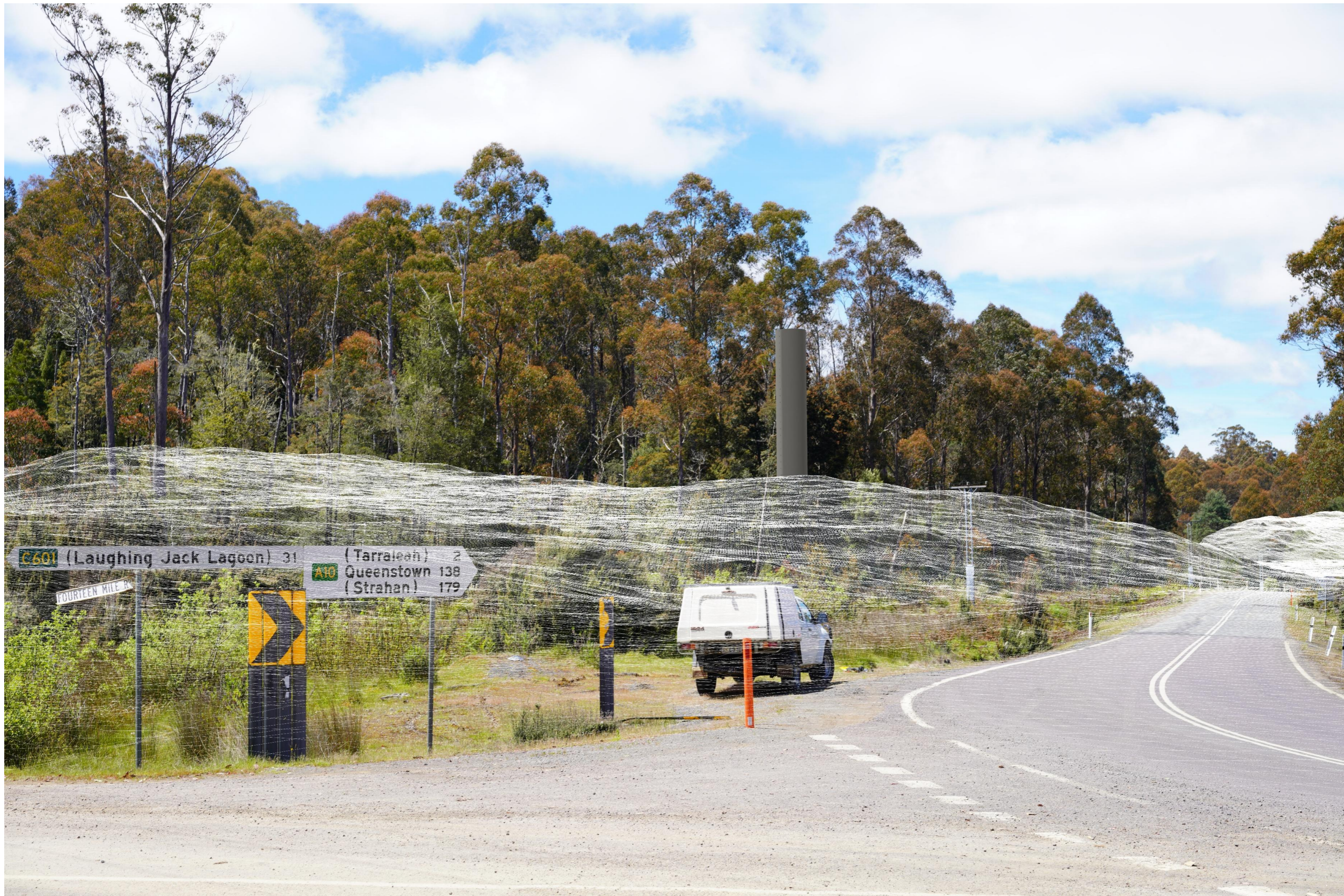
MPP – Tarraleah Surge Tower wireframe on DEM View from Fourteen Mile Road & Lyell Highway intersection
