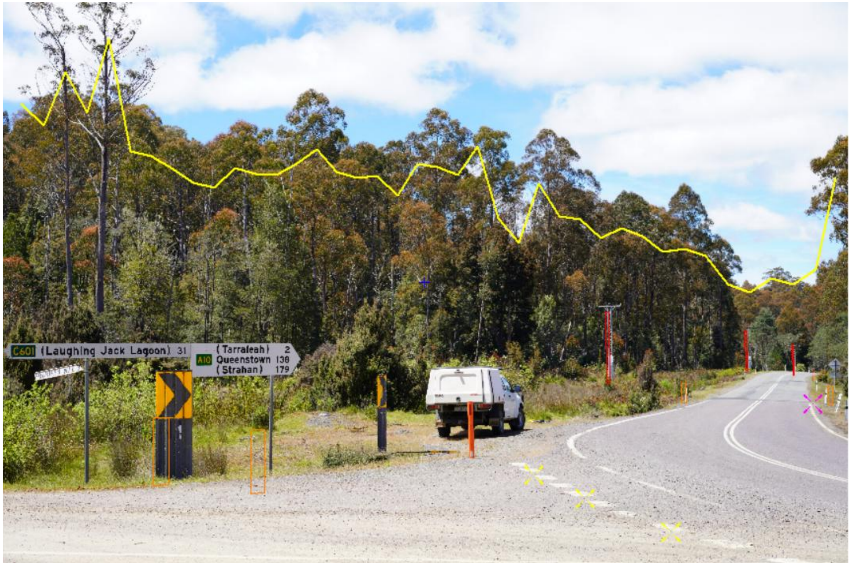
MPP – Tarraleah Surge Tower Calibration View from Fourteen Mile Road & Lyell Highway intersection
