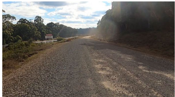
Figure 7: Butlers Gorge Road - evidence of coarse aggregate surface (-42.276, 146.326)
