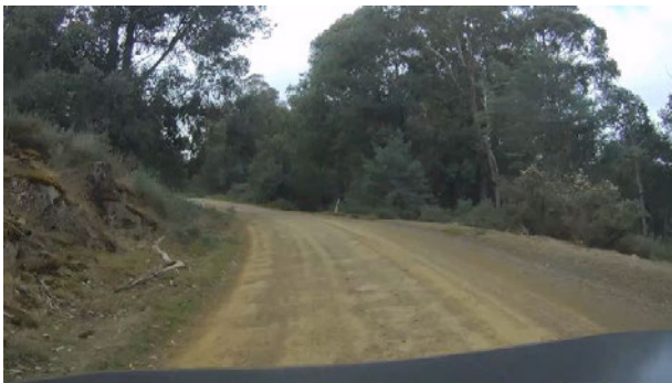
Figure 12: Victoria Valley Road - evidence of minor corrugations (-42.188, 146.511)
