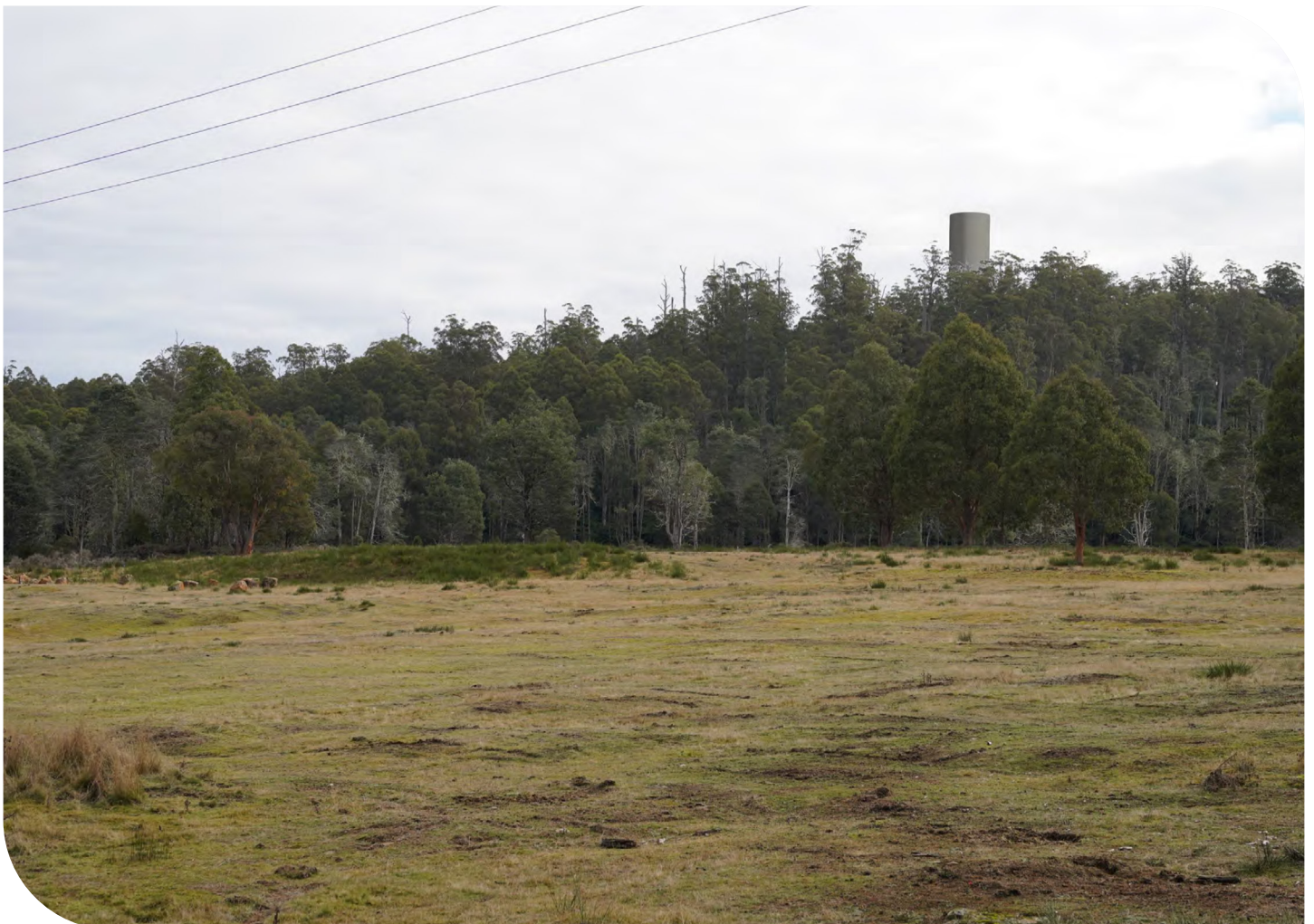
Tarraleah Surge Tower Visual Simulation Oldina Drive – view from beside penstocks
