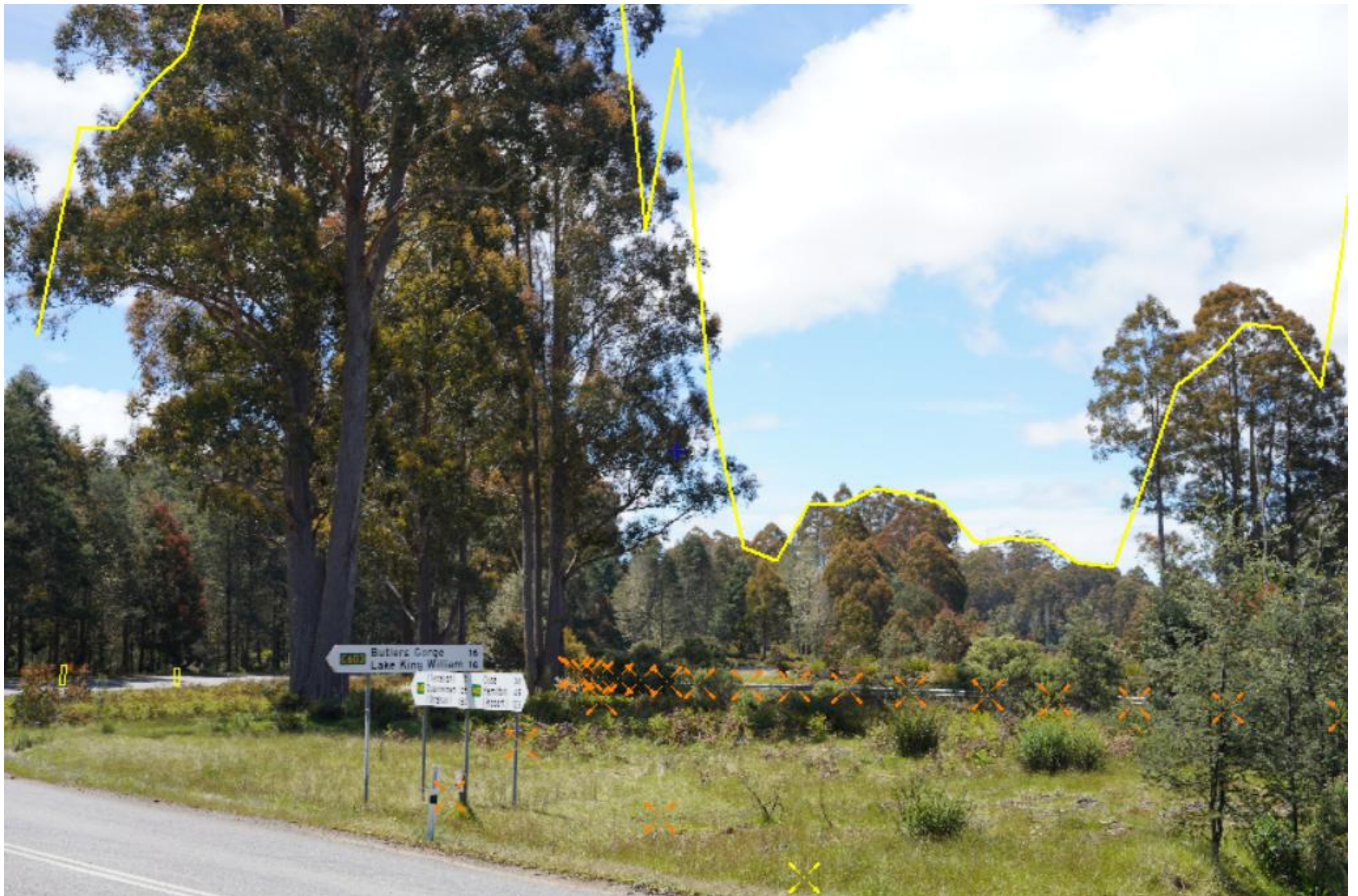
MPP – Tarraleah Surge Tower Calibration View from Butlers Gorge Road & Lyell Highway intersection
