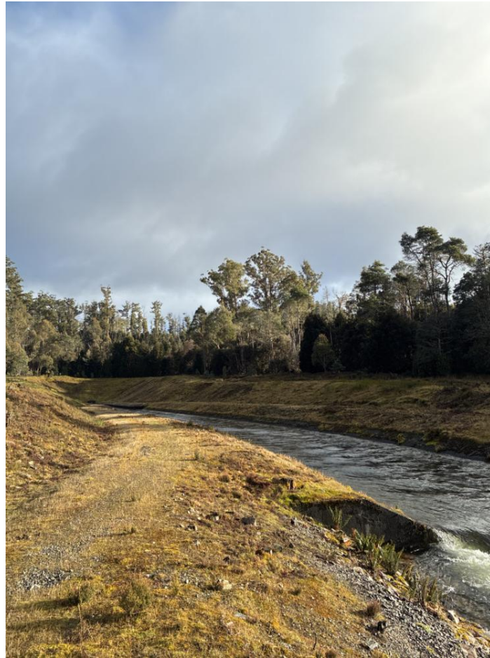
Figure 4.4: Water quality sampling site SW-P1 (161.26) located at the exit point of Canal No. 2 tunnel
