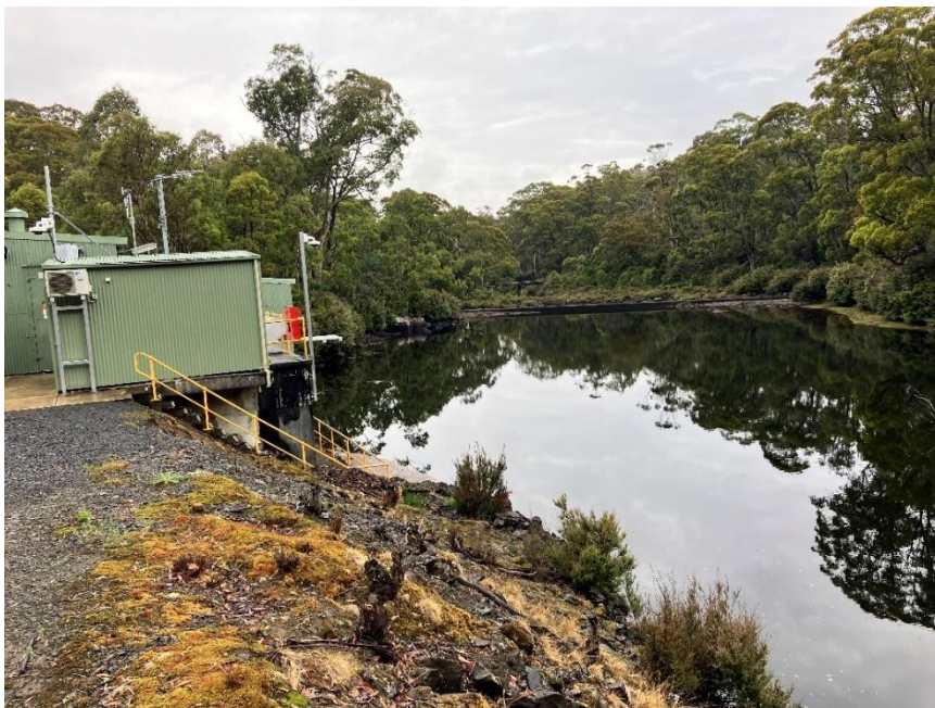
Figure 6.10: The impounded River Derwent at Derwent Pumps Weir, located 6 km downstream from Clark Dam. Pump infrastructure (at left) pumps water to No. 2 Canal via pipeline.
