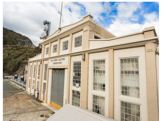
Figure 25: Tarraleah Power Station
