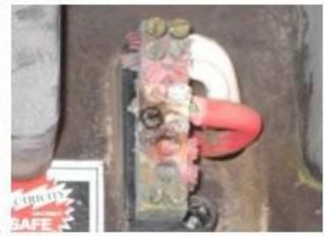
Poor termination / corrosion on link
