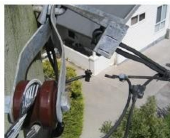
Broken service neutral at pole
