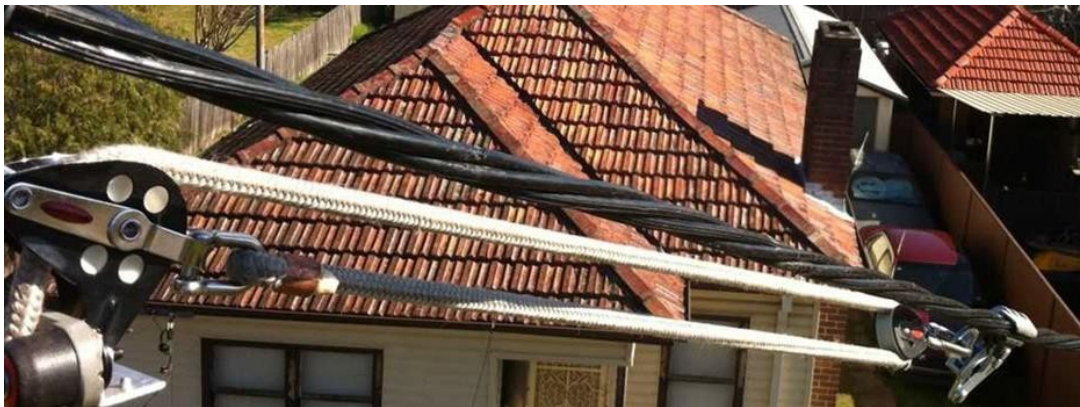
Typical cable strain grip and come along on ABC service
