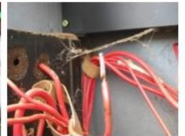
Termination loose - over heating
