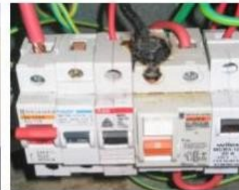
Loose RCD connection
