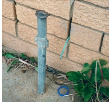
Example of defective earth connection
