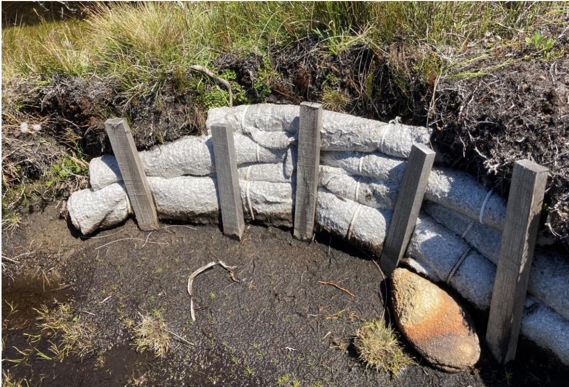
Figure 11 Small coir logs reducing frost heave and supporting a deflated pool at Pine Marsh Bay, Lake Mackenzie
