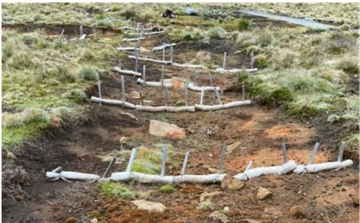
Figure 12 Small coir logs acting as weirs to slow overland flow in area of gully erosion at Ritters Plain, Lack Mackenzie. This is the proposed treatment for the gully erosion on the lake bed adjacent to the dunes.
