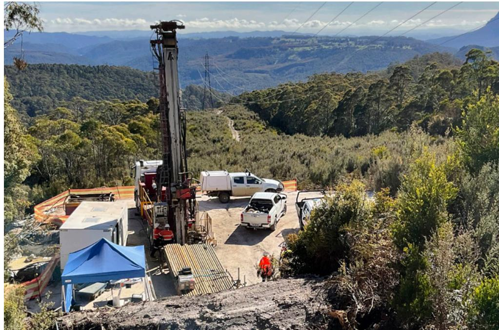
We've now completed our geotechnical investigations to find out more about the ground conditions at the upper storage site. The data from the investigations helps us to better understand the surface and underground conditions and the materials present at the site. We had up to three drilling rigs completing our geotech program between August 2023 and July 2024.
