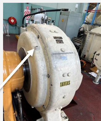
Anchor point eye bolt was screwed in to
