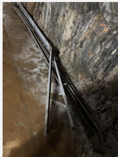
6m length removed cable tray
