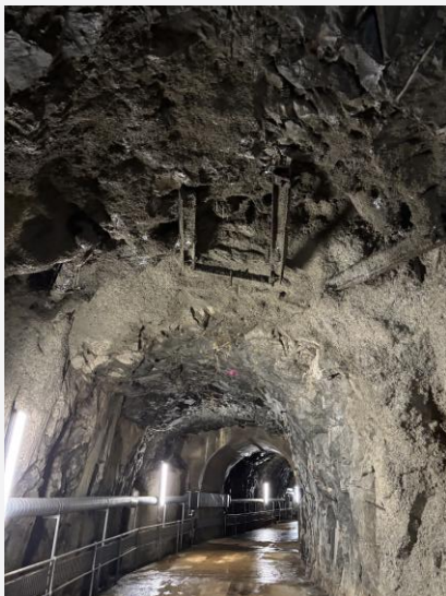
Ceiling of tunnel where cable trays were installed
