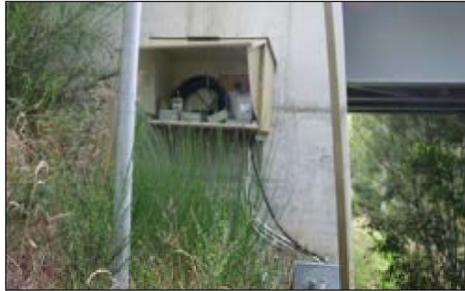
Figure F.2: Judbury flood gauge located on the right bank (looking downstream) on the downstream abutment (0m at the gauge = 10.91m AHD)
