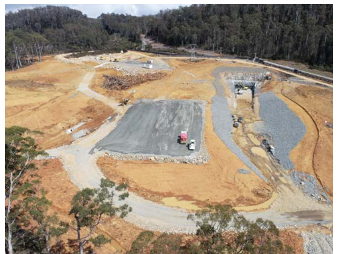
Above: An aerial view of the downstream tunnel portal of the Lake King William tunnel that will commence construction in early 2024. The 1km tunnel will link the new intake at Lake King William to a future new water conveyance. Site rehabilitation is now underway.
