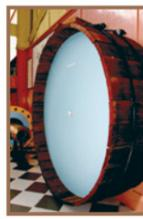
Four wooden pipes were used - each pipe was 2.4 kms. Steel was scarce during the war so wood was used for pipes when the pressure was less than 200 pounds per square inch (psi). At the power station the pressure was 500 psi and required steel.
