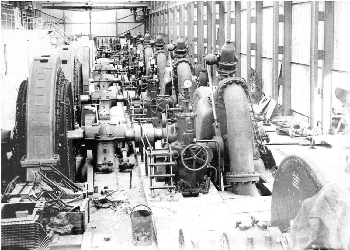
**Figure 2.4** Construction of the extension to Waddamana A looking southwest (Hydro Tasmania).
