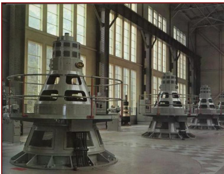
Figure 2.14: Tungatindah Turbine Hall c. 1961, showing exciters and original checked floor colour scheme.<sup>86</sup>
