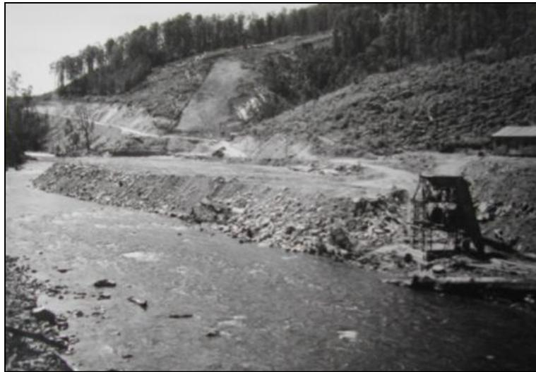
**Figure 2.4: The Power Station site towards the end of 1949. Note the concrete plant in the right of the photo and the wooden hut above it.<sup>31</sup>**
