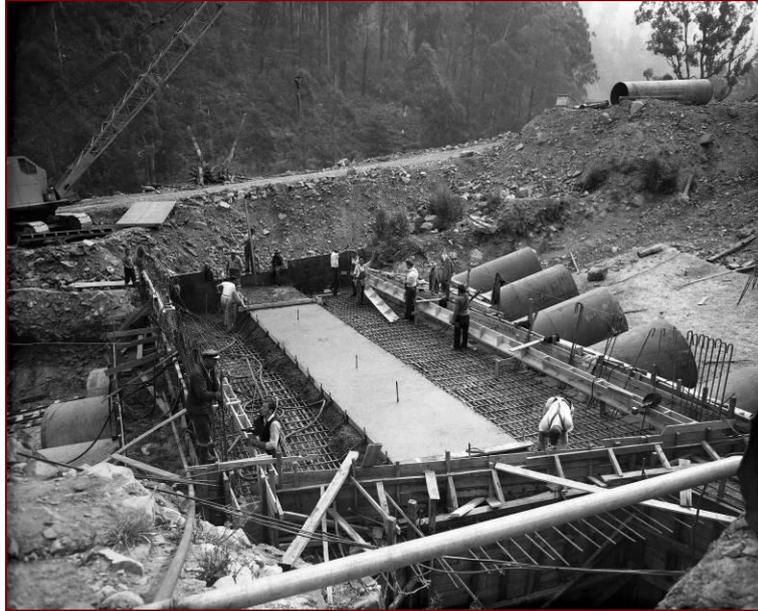
Figure 2.7: Placing concrete in anchor for the Tungatinah penstocks.<sup>54</sup>
