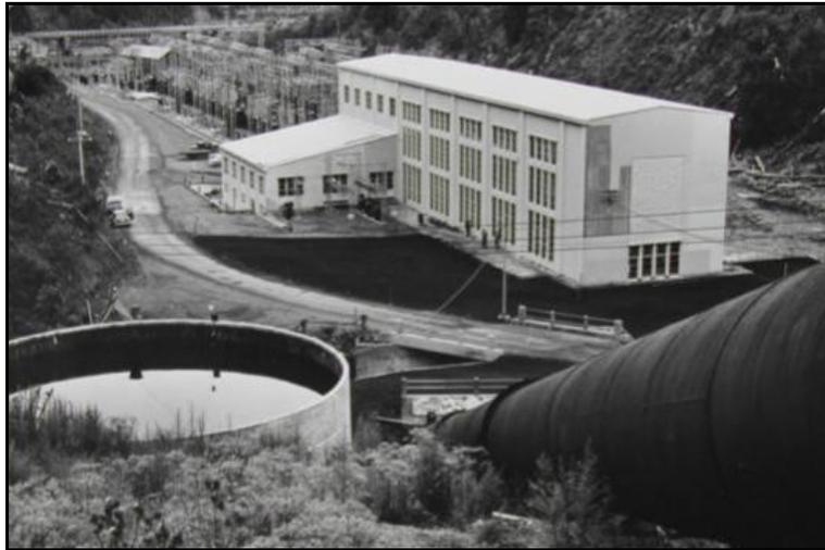
**Figure 2.10: Tungatinah Power Station (24/04/1955, shortly before the official opening. Note the cooling water tank and penstocks in the foreground and the painting nearing completion.<sup>68</sup>**
