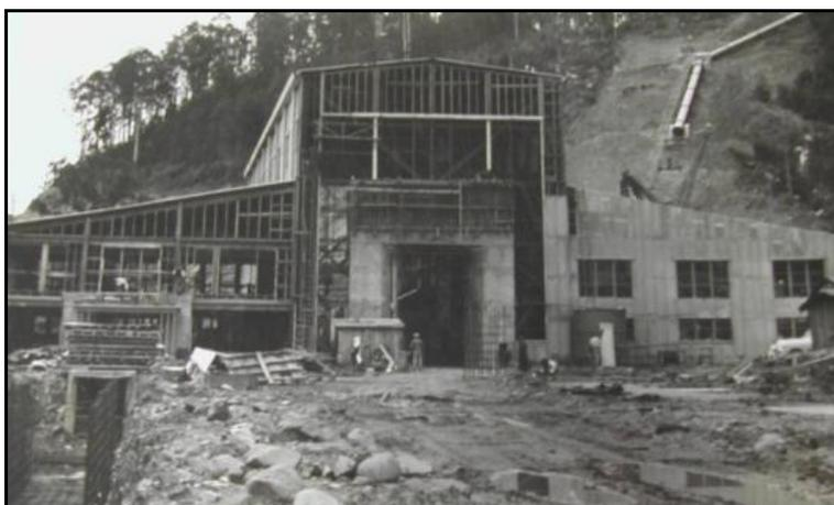
Figure 2.9: The southern end of the Power Station building (09/02/1952). Note the single penstock under construction in the top right-hand corner.<sup>67</sup>
