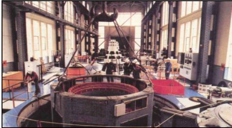
**Figure 2.17: Maintenance on an alternator at Tungatinah, c.1985. Note the uniform blue floor.<sup>101</sup>**
