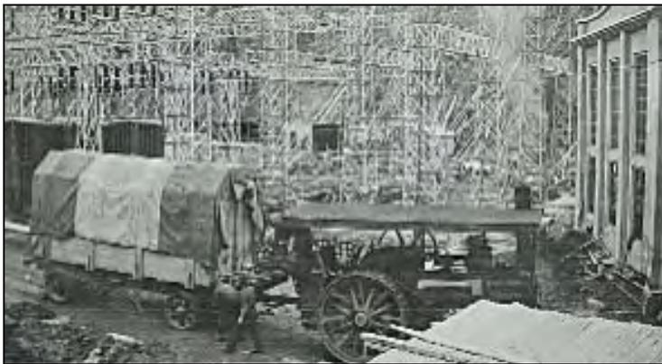
**Figure 8: 1937 photograph of plant being delivered by traction engine to the Tarraleah Power Station in 1937 (Cyril Young Collection —AOT, NS19388/142).**
