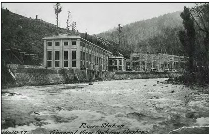
**Figure 18: View of power station from down stream showing stone walling along the river bank (HEC collection).**
