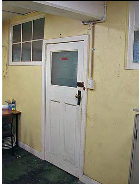
**Figure 82: View of room showing painted internal timber work, standard first floor door, modern light switch and conduits and the building's structural framing expressed in the ceiling. This is typical of the utilitarian spaces of the first floor.**
