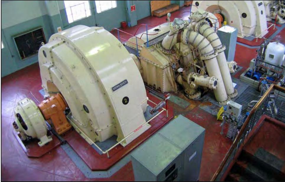
**Figure 97: Overview of Boving & Co machine #2. Picture from L; Exciter, alternator, turbine & spears.**
