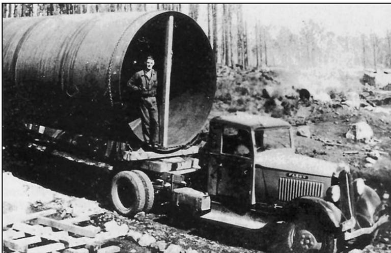
**Figure 25: Section of 102 inch pipe being transported to hilltop penstock (HEC collection, reproduced in Marwood, p. 48).**
