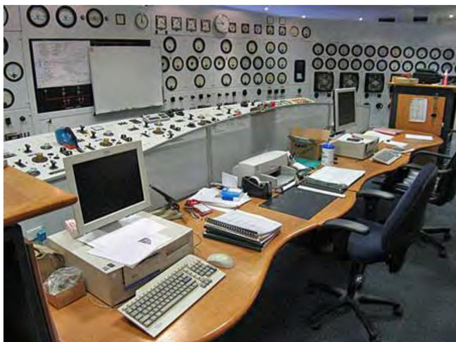
**Figure 67: View of control room showing various stages in control technology including the 1937 control panel, the control bench board and the modern and office desk and computers.**
