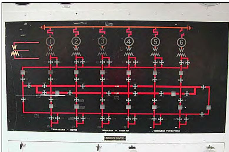
**Figure 65: Redundant circuit diagram for the six generating machines, located on the main control panel.**
