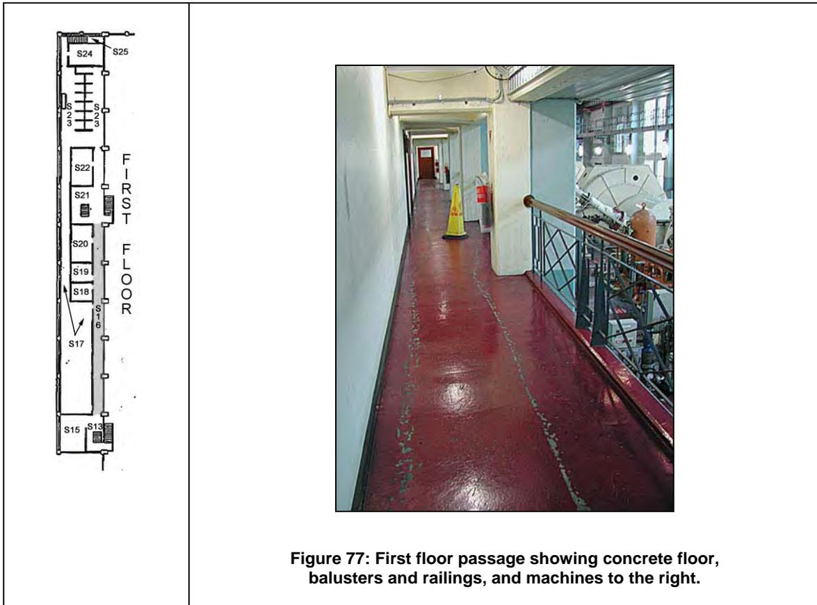
**Figure 77: First floor passage showing concrete floor, balusters and railings, and machines to the right.**
