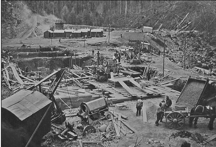
**Figure 13: View of power station site in 1934/35 during earlier phase of construction showing the use of manual, horse driven and machine power (Cyril Young Collection, AOT - NS1938/138).**
