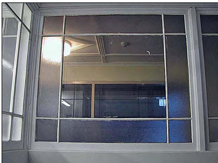
**Figure 53: Internal window between S4 and passageway showing drawn glass central pane surrounded by *Belgian stippolite* perimeter panes. Note also the window to S3, the ceiling detail of the passageway and the smoke detector. The window arrangement is typical of the second floor internal windows throughout unless otherwise noted.**
