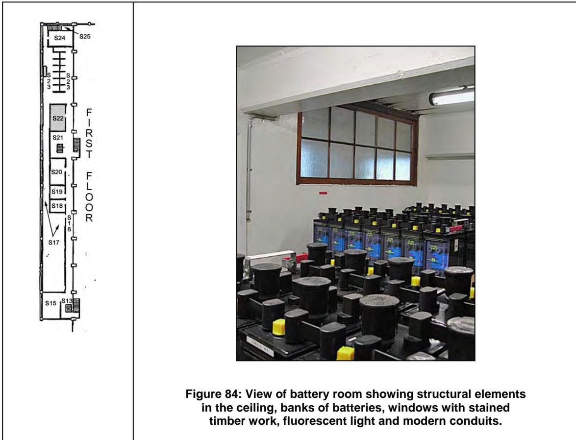
**Figure 84: View of battery room showing structural elements in the ceiling, banks of batteries, windows with stained timber work, fluorescent light and modern conduits.**
