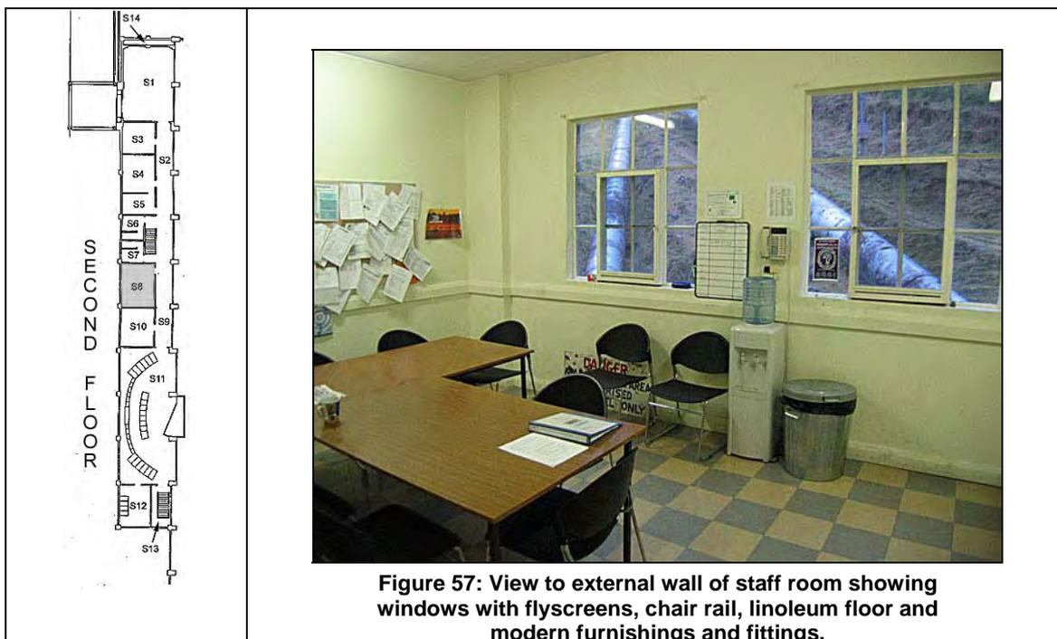
**Figure 57: View to external wall of staff room showing windows with flyscreens, chair rail, linoleum floor and modern furnishings and fittings.**
