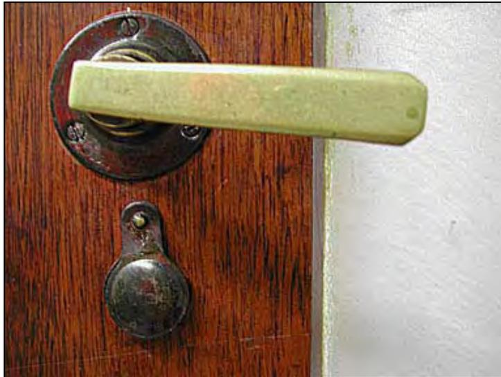
**Figure 51: Detail of original door furniture in S4. This is typical of many door handles found in the internal room doors on the second floor of the building.**
