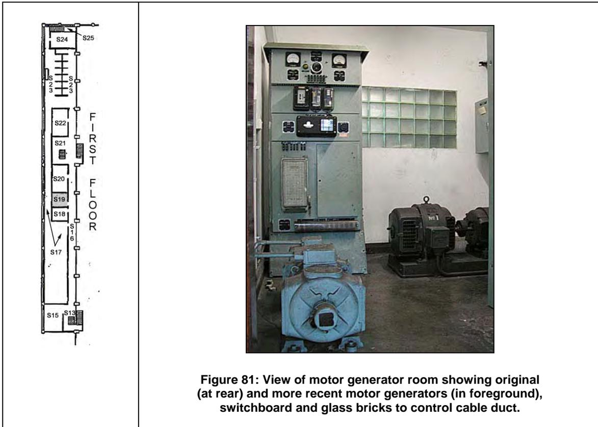
**Figure 81: View of motor generator room showing original (at rear) and more recent motor generators (in foreground), switchboard and glass bricks to control cable duct.**
