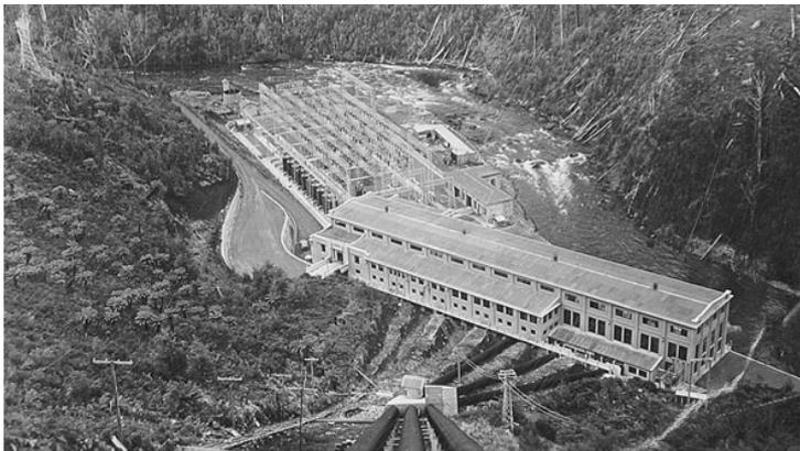
**Figure 17: View of power station and switchyard soon after opening showing penstock, excavations for three more penstocks and the workshop/store adjacent to the switchyard (HEC collection).**
