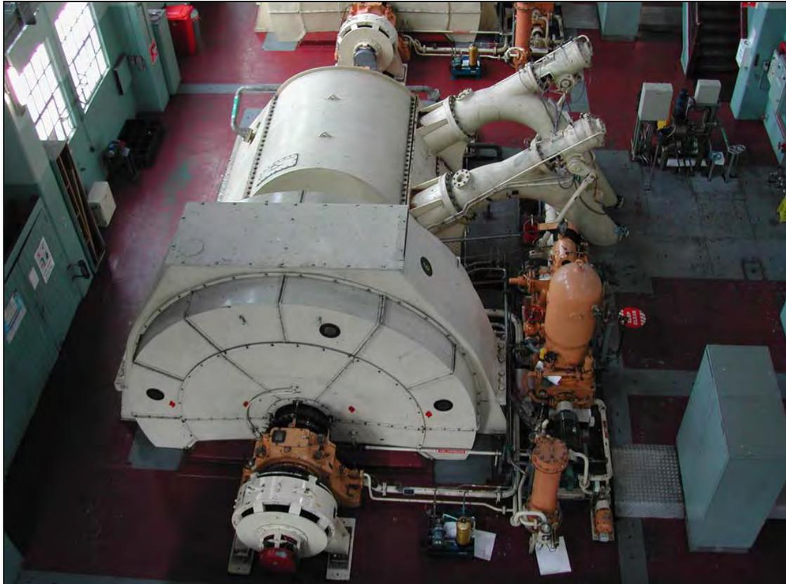
**Figure 98: Overview of English Electric Co machine #6 showing, exciter, turbine & spears, governor & alternator.**
