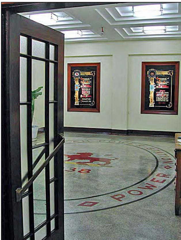
Figure 43: View of vestibule from S2 showing door to S2, Art Deco ceiling, terrazzo floor and stained glass windows.
