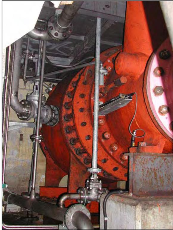
Figure 99: Sub-floor view showing main inlet valve to English Electric Co machine #5.
