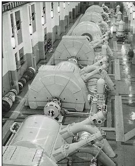
**Figure 33: Interior of power station with six machines. The three original Boving Ltd machines are in the background with the three newer English Electric Co machines in the foreground. (HEC collection).**
