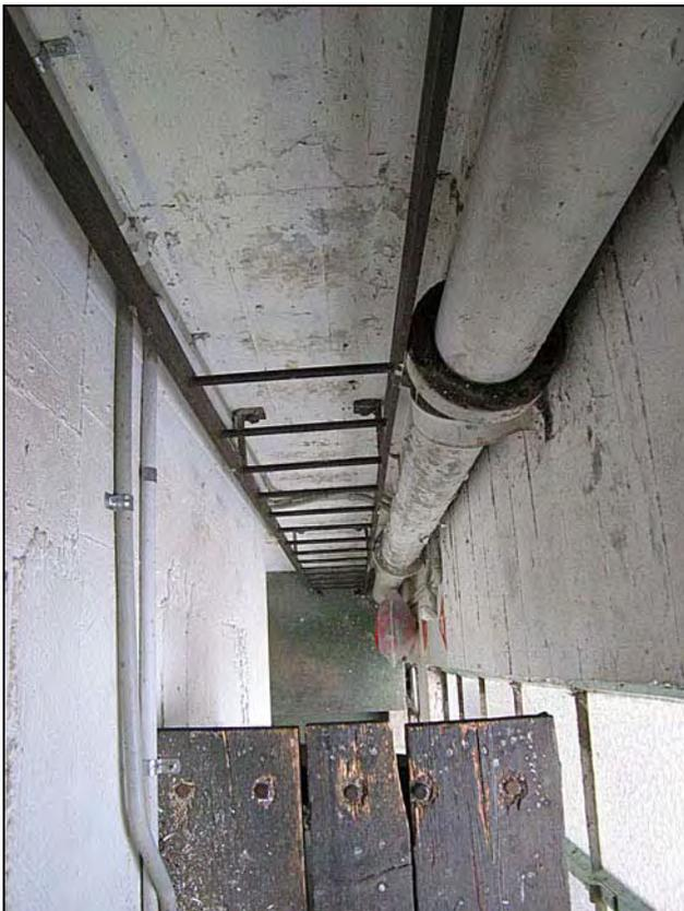
**Figure 74: Wall mounted iron ladder used to access maintenance space behind memorial stained glass windows. Note the downpipe, the timber plank flooring and the evidence of formwork erected when pouring concrete for the building.**
