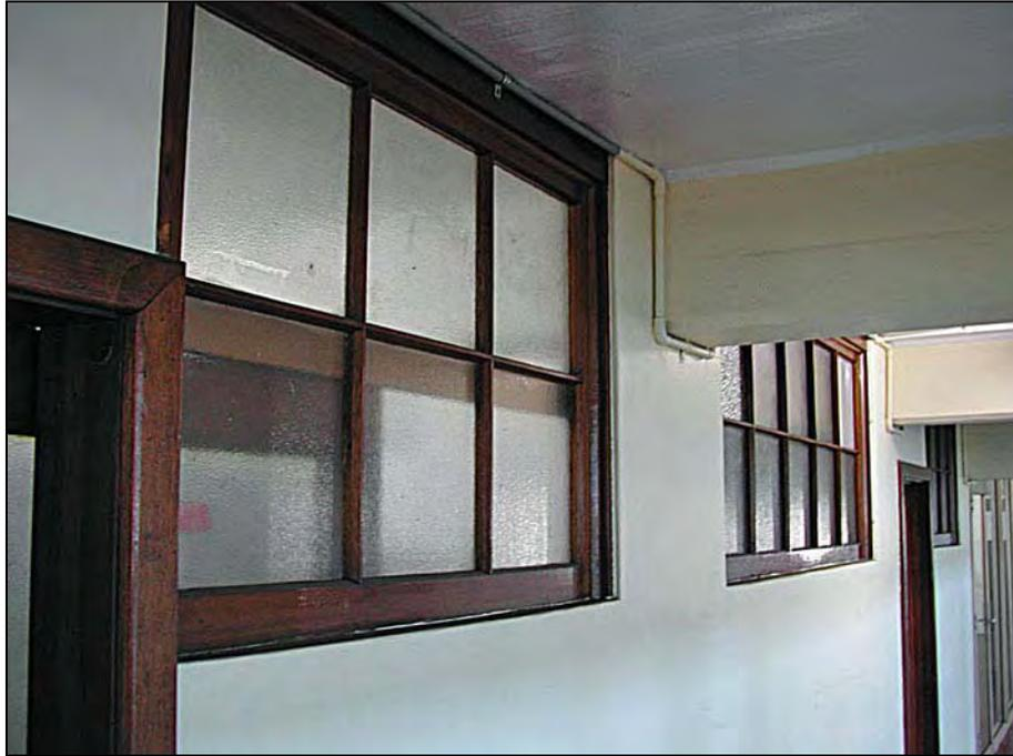
**Figure 78: Detail of internal windows to S19 & S20 from the first floor passage. Note the concrete beams and electrical conduits.**
