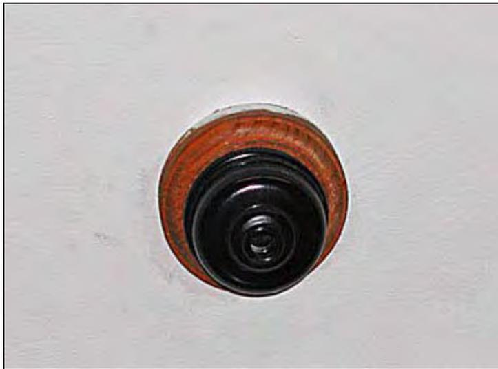
**Figure 52: Original timber and bakelite light fitting on ceiling of S4. This type of fitting is now rare inside the building.**
