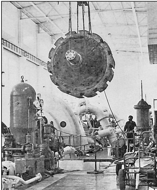
**Figure 40: Number 4 rotor being lifted into position by the overhead crane following rewinding in 1979 (*Cross Currents*, December 1979, p. 9).**
