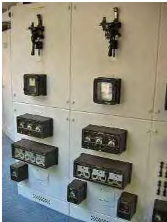
**Figure 66: Relays and controls for the auxiliary generators. This is part of the only fully intact original generator system in the power station.**
