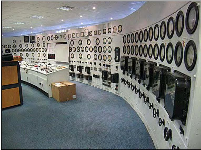
**Figure 63: Main control panel in Tarraleah control room, with the original bench board in front and c1980s console to the left. Much of the instrumentation is now redundant.**
