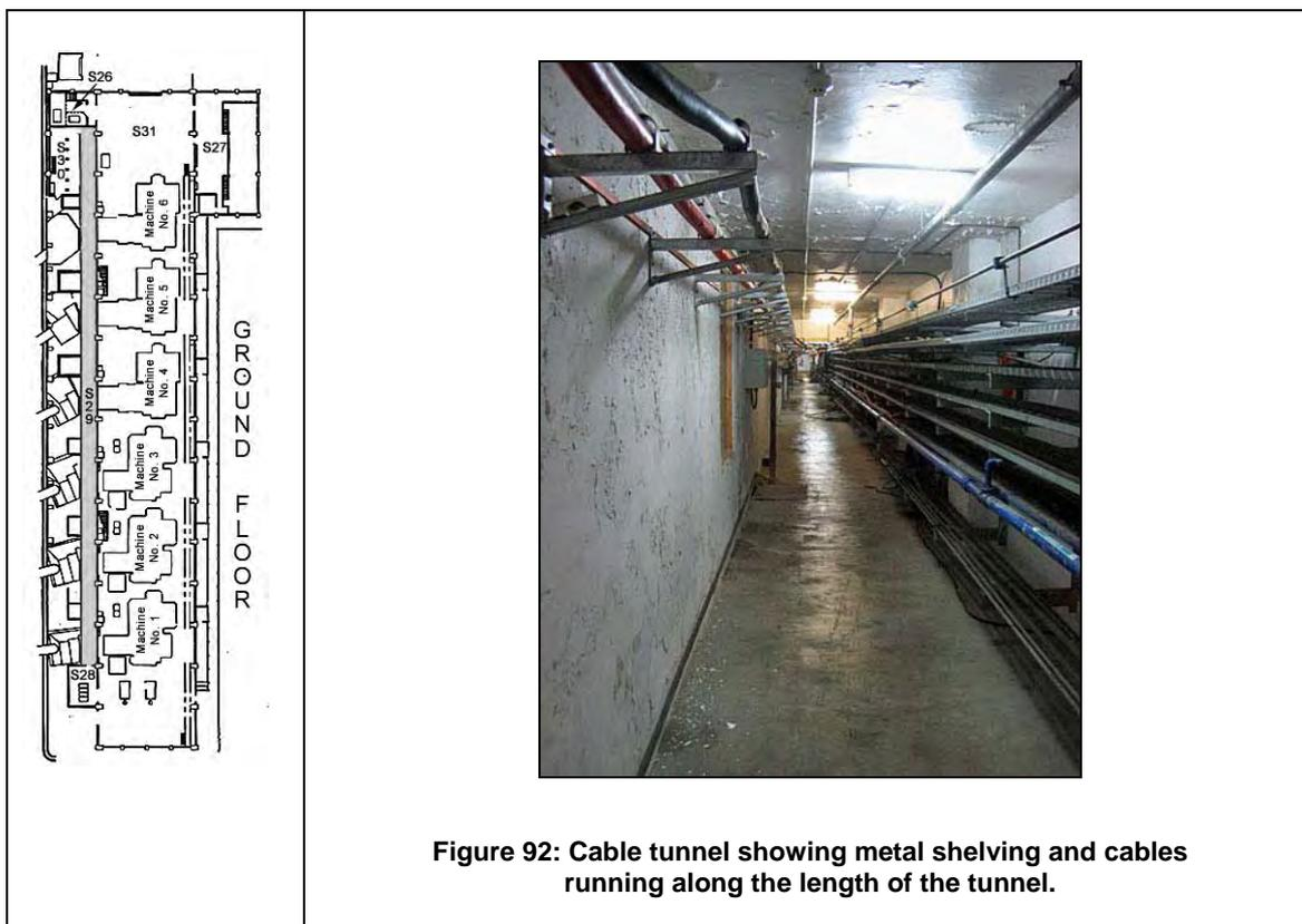
Figure 92: Cable tunnel showing metal shelving and cables running along the length of the tunnel.
