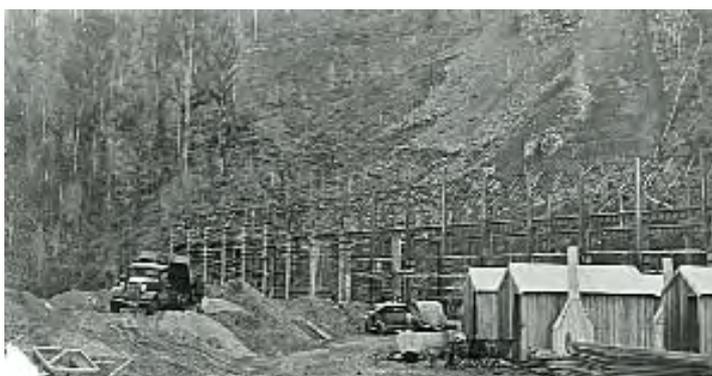
**Figure 6: c1935 view of steel frame of power station erected with hillside behind cleared for penstock and temporary vertical board huts in foreground (HEC collection).**
