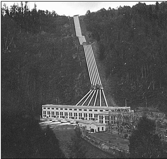
**Figure 35: View of the power station in late 1950s. Note that the wing extending towards the river from the north-eastern end of the workshop has been removed (HEC collection).**
