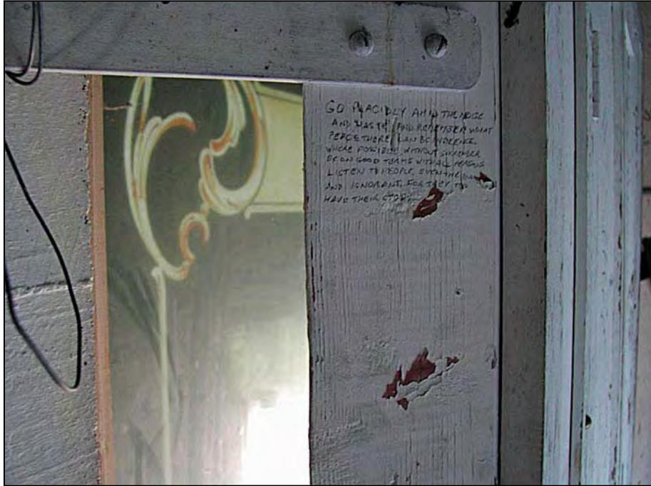
**Figure 73: Detail of screen, fixings, graffiti and memorial stained glass windows. Note evidence of formwork used in the construction of the concrete walls.**
