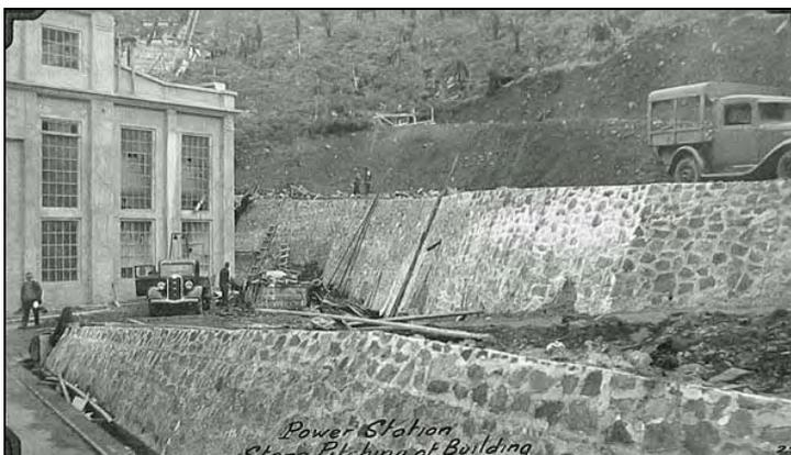
**Figure 15: Stone retaining walls built at the front of the power station. Similar walls were built along the river bank (HEC collection).**
