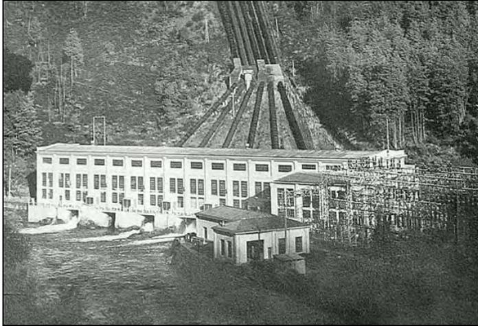
**Figure 34: View of power station in 1950s showing the location and layout of the workshop adjacent to the switchyard and the six hillside penstocks - compare with figure 35 for changes to workshop (HEC collection).**
