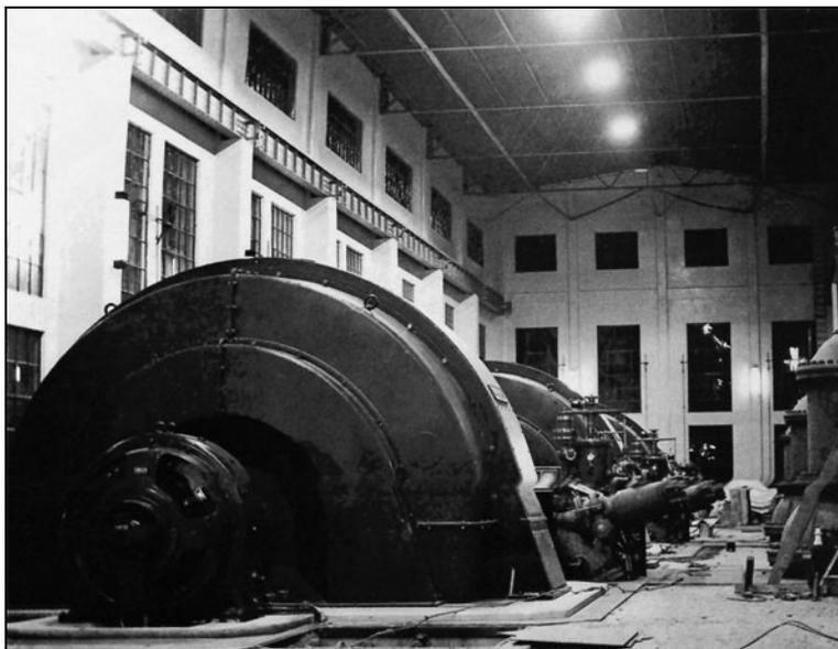
Figure 20: Three Boving & Co. machines installed at Tarraleah in 1937 (HEC photographic collection, reproduced in Lupton, p. 133).
