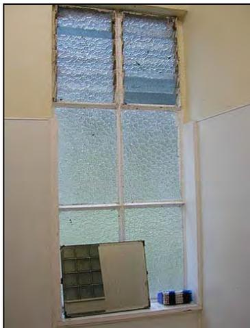
**Figure 56: External window in S7. Note Arctic glass panes and louvres.**
