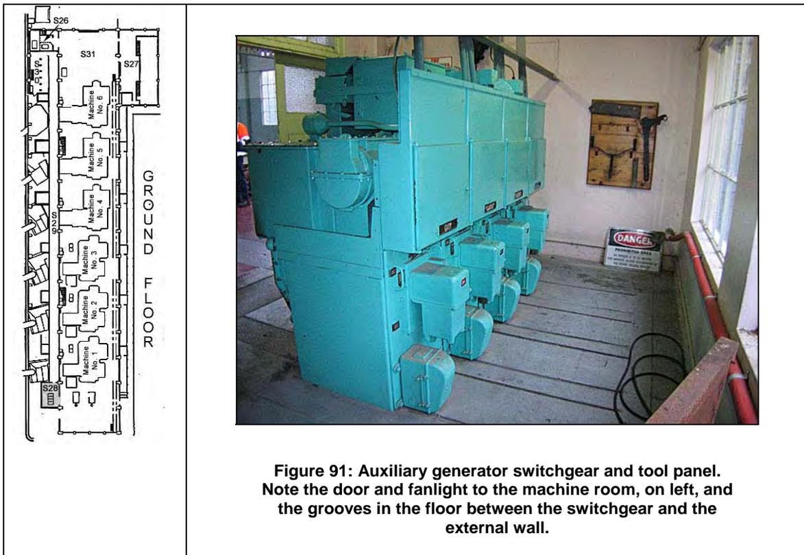
**Figure 91: Auxiliary generator switchgear and tool panel. Note the door and fanlight to the machine room, on left, and the grooves in the floor between the switchgear and the external wall.**
