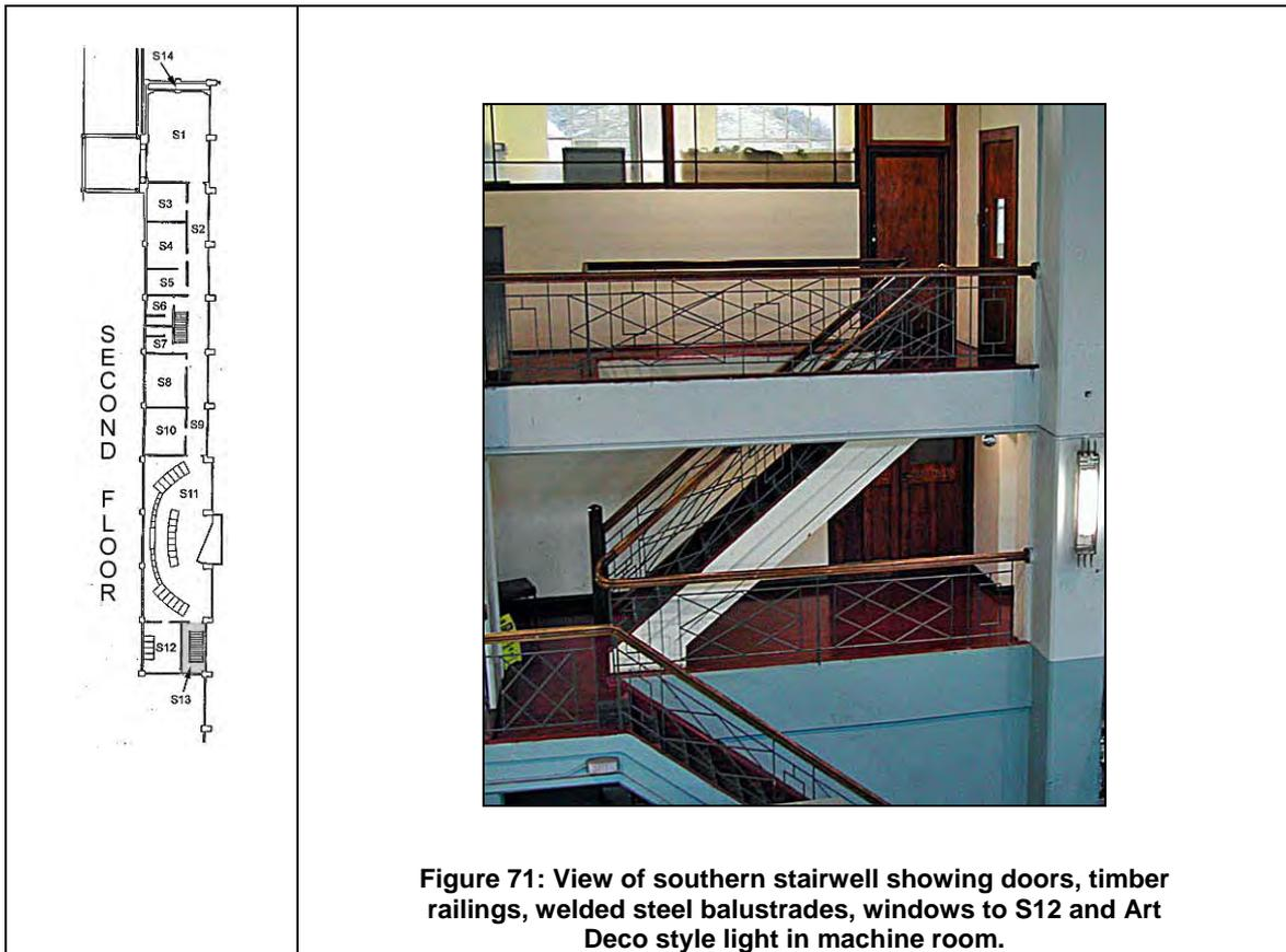
**Figure 71: View of southern stairwell showing doors, timber railings, welded steel balustrades, windows to S12 and Art Deco style light in machine room.**
