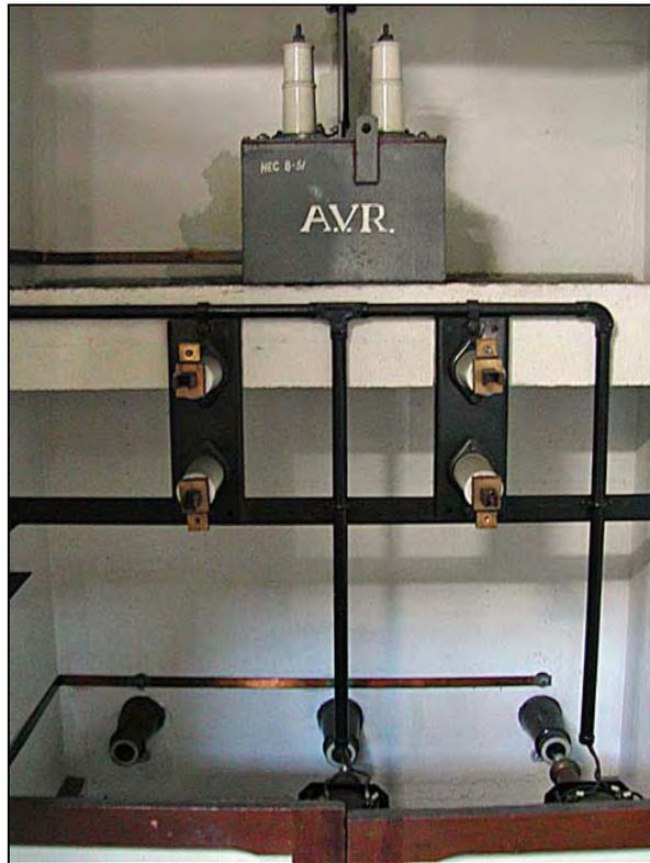
Figure 86: Remnant electrical equipment in transformer cubicle.
