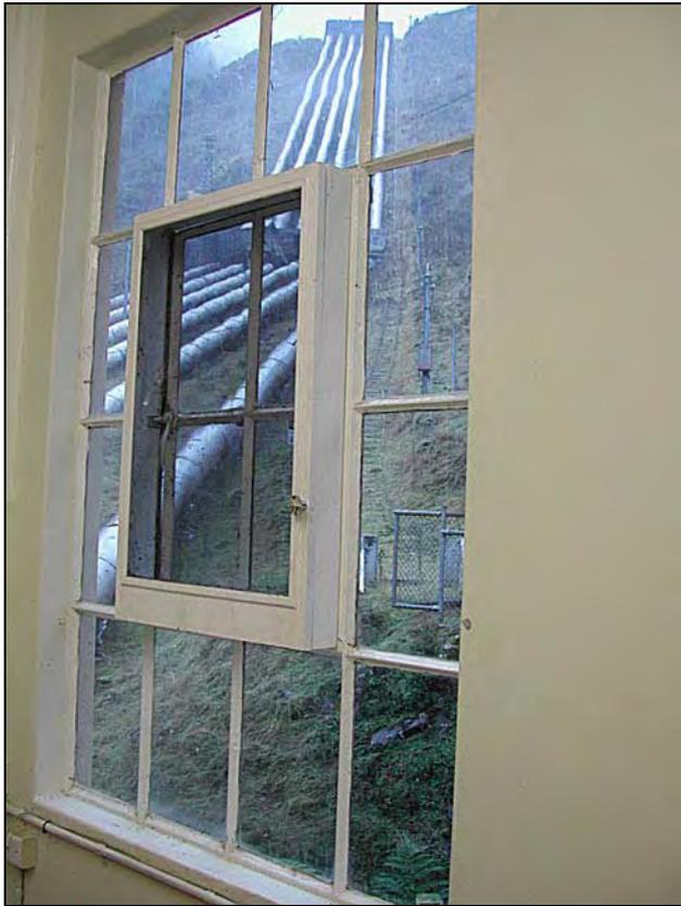
**Figure 49: External window in team leader’s office showing the centrally located opening casement and retro fitted timber framed insect screen. This window arrangement, with variation to the numbers of panes, is typical throughout the building.**
