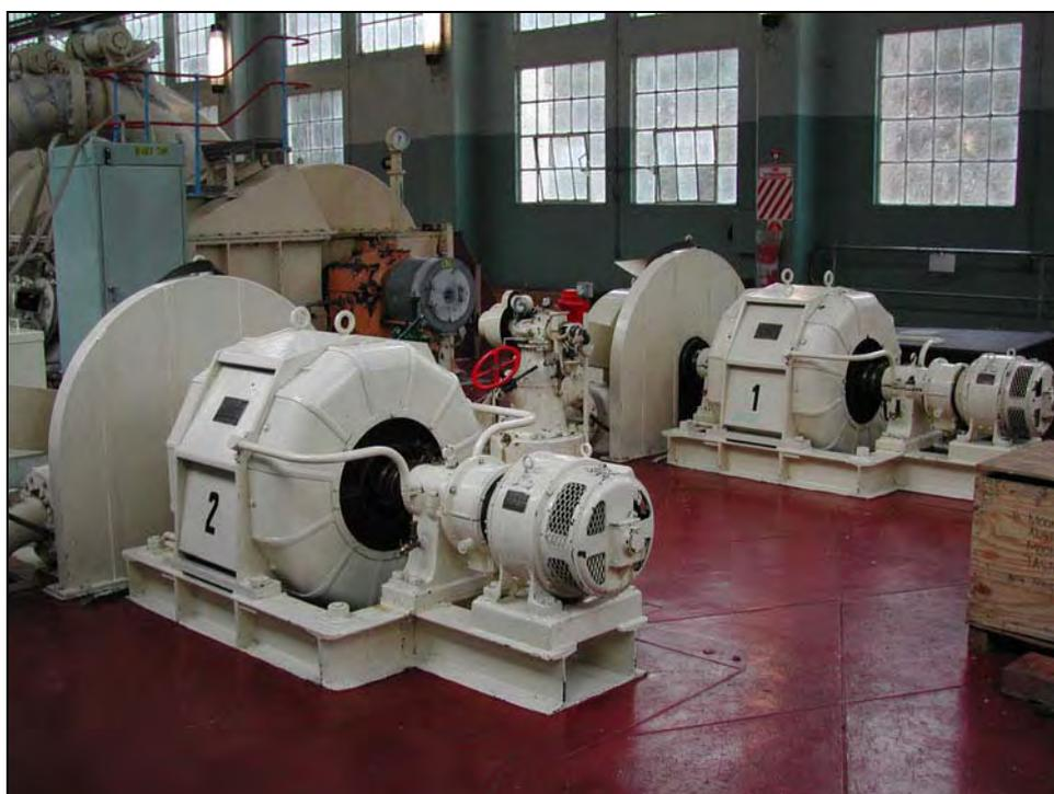
Figure 95: View of auxiliary (or 'house supply') generators 1 & 2. Exciters and turbines pictured.
