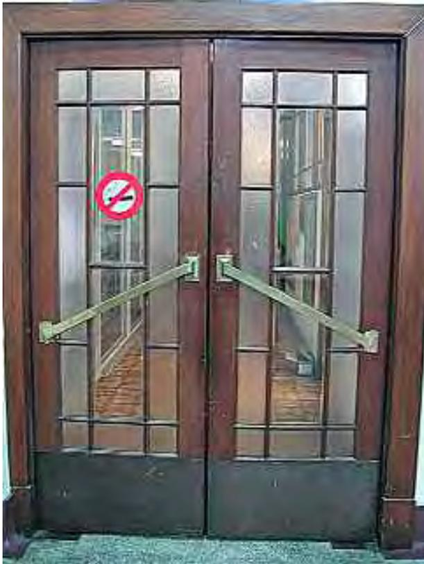
**Figure 46: View of door between S1 and S2 showing timber and brass detailing, and both the plain and stipplite glass panels. Apart from the No Smoking sticker this door is identical to the door between S2 and S9.**
