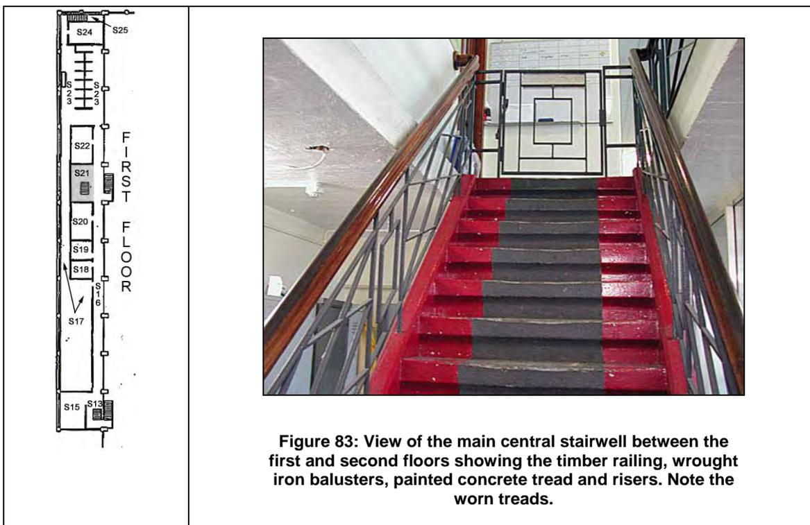
**Figure 83: View of the main central stairwell between the first and second floors showing the timber railing, wrought iron balusters, painted concrete tread and risers. Note the worn treads.**
