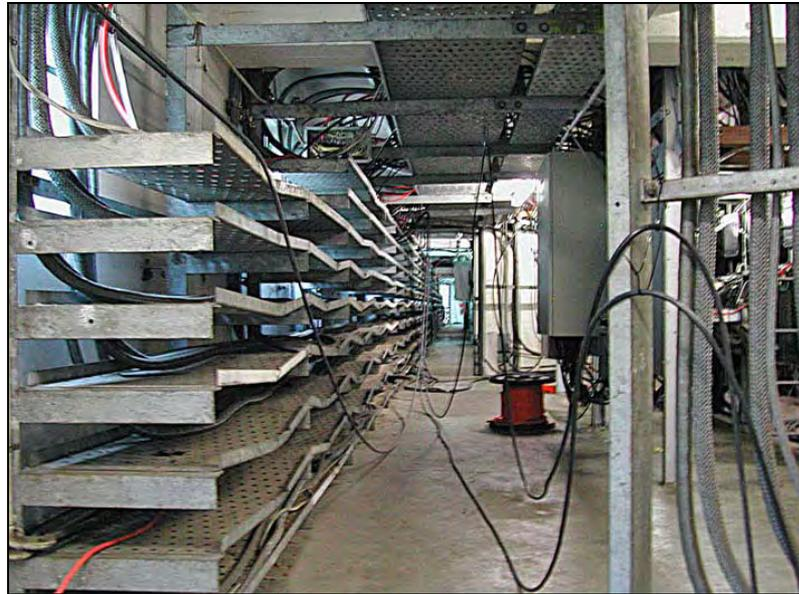
**Figure 79: View of former terminal room showing shelves of cables leading to and along the length of the control cable duct.**
