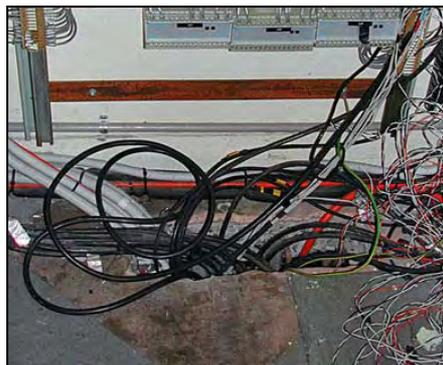
**Figure 62: Hole cut in concrete in SW corner of floor of S10 to allow passage of cables after the room was converted to a communications room.**
