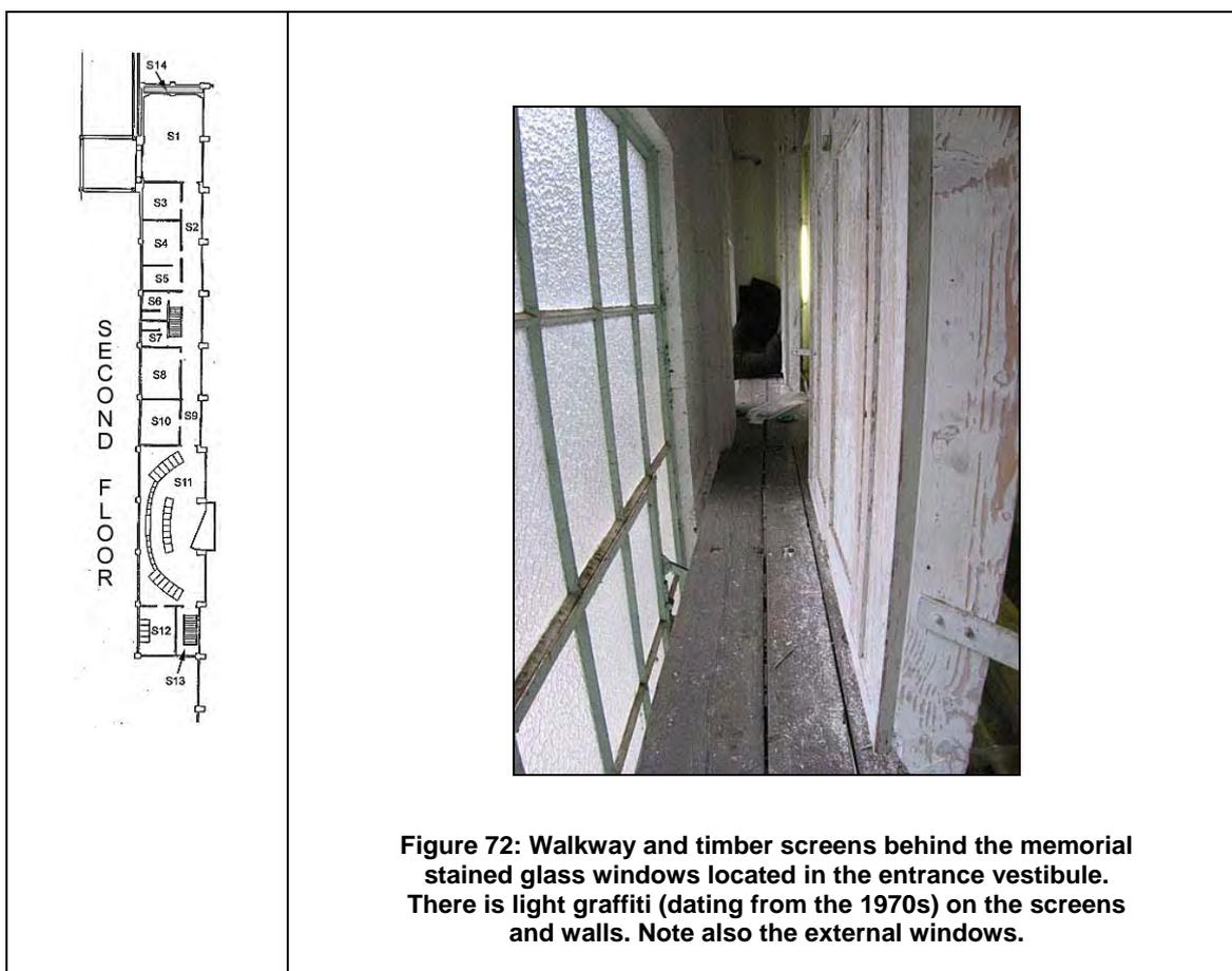
**Figure 72: Walkway and timber screens behind the memorial stained glass windows located in the entrance vestibule. There is light graffiti (dating from the 1970s) on the screens and walls. Note also the external windows.**
