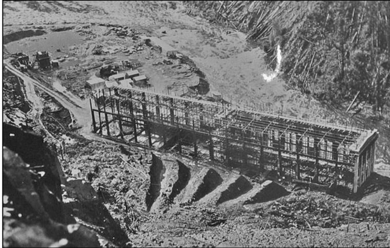
**Figure 28: Power station under construction showing the excavations for the first five penstocks adjacent to the station. The sixth trench was excavated soon afterwards (HEC collection).**
