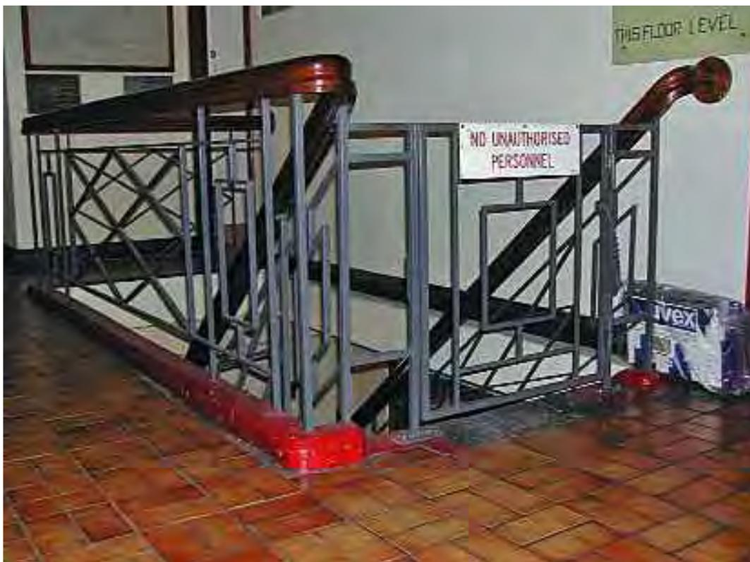
Figure 45: Central stairwell to first and ground floors showing late twentieth century tiled flooring and Art Deco painted welded steel balusters and gate, and varnished timber railing.
