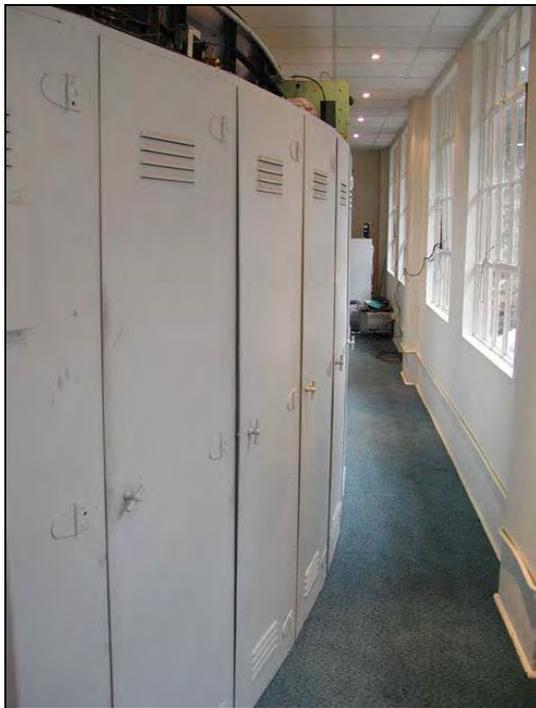
**Figure 64: Rear of control cabinet showing metal doors with original handles to access electronic circuitry in the board. Note the windows in the external wall.**
