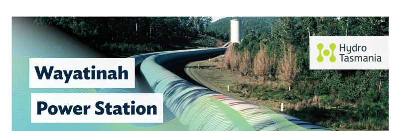
Wayatinah Power Station is the sixth station on the Lower Derwent / Nive Scheme. The station was commissioned in 1957 and houses three machines comprised of English Electric generators, coupled to English Electric Francis turbines in concrete embedded spiral casings.
