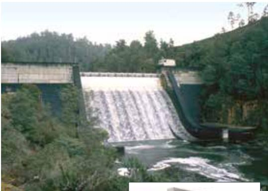
*The Liapootah Dam is a concrete gravity dam 40m high*
