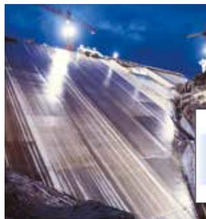
*The largest concrete-faced rockfill dam in Tasmania is the Reece Dam, which is 122m high and contains more than 2.6 million cubic metres of fill*
