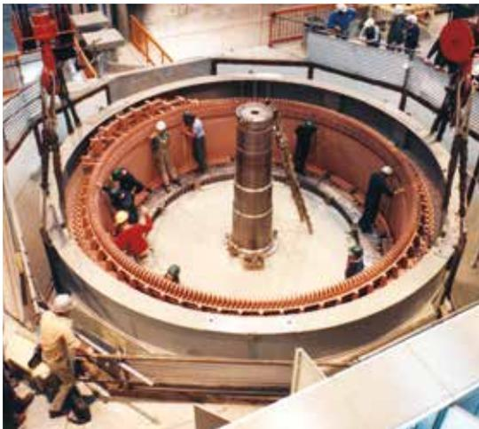
The coils of conductor in the outer section of the generators at Gordon Power Station
