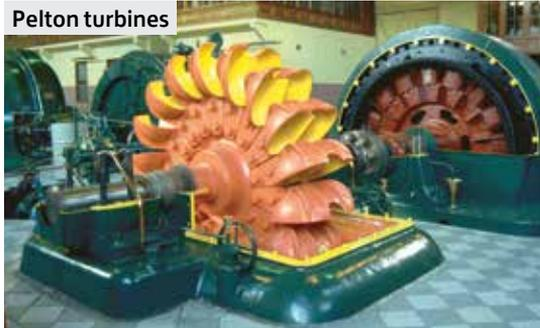
Pelton turbines operate when one or more jets of water under extremely high pressure are squirted from nozzles onto buckets on the edge of a circular wheel.
