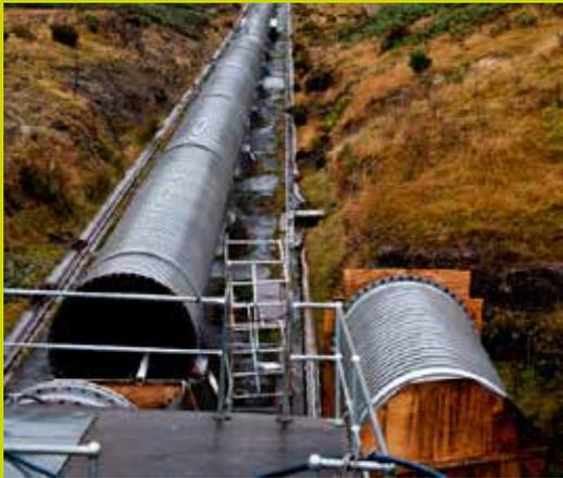
Removing a section of the Poatina penstock to gain internal access
