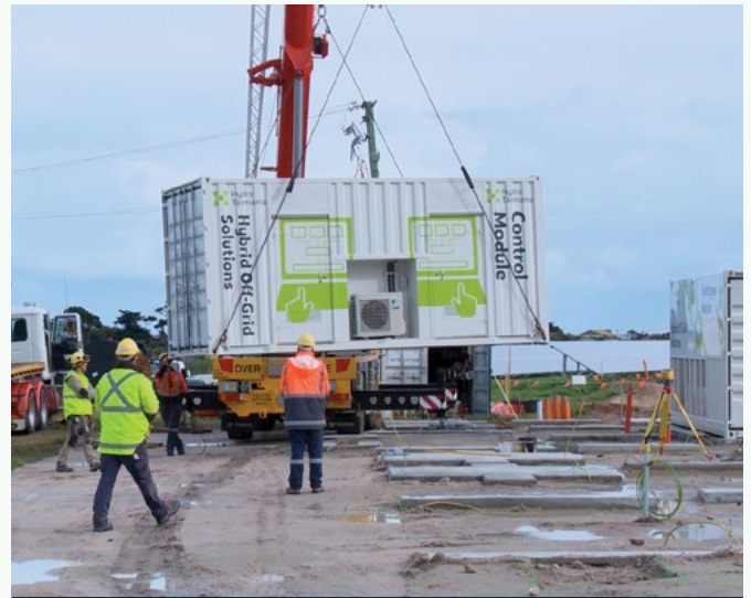
Placing containerised equipment
