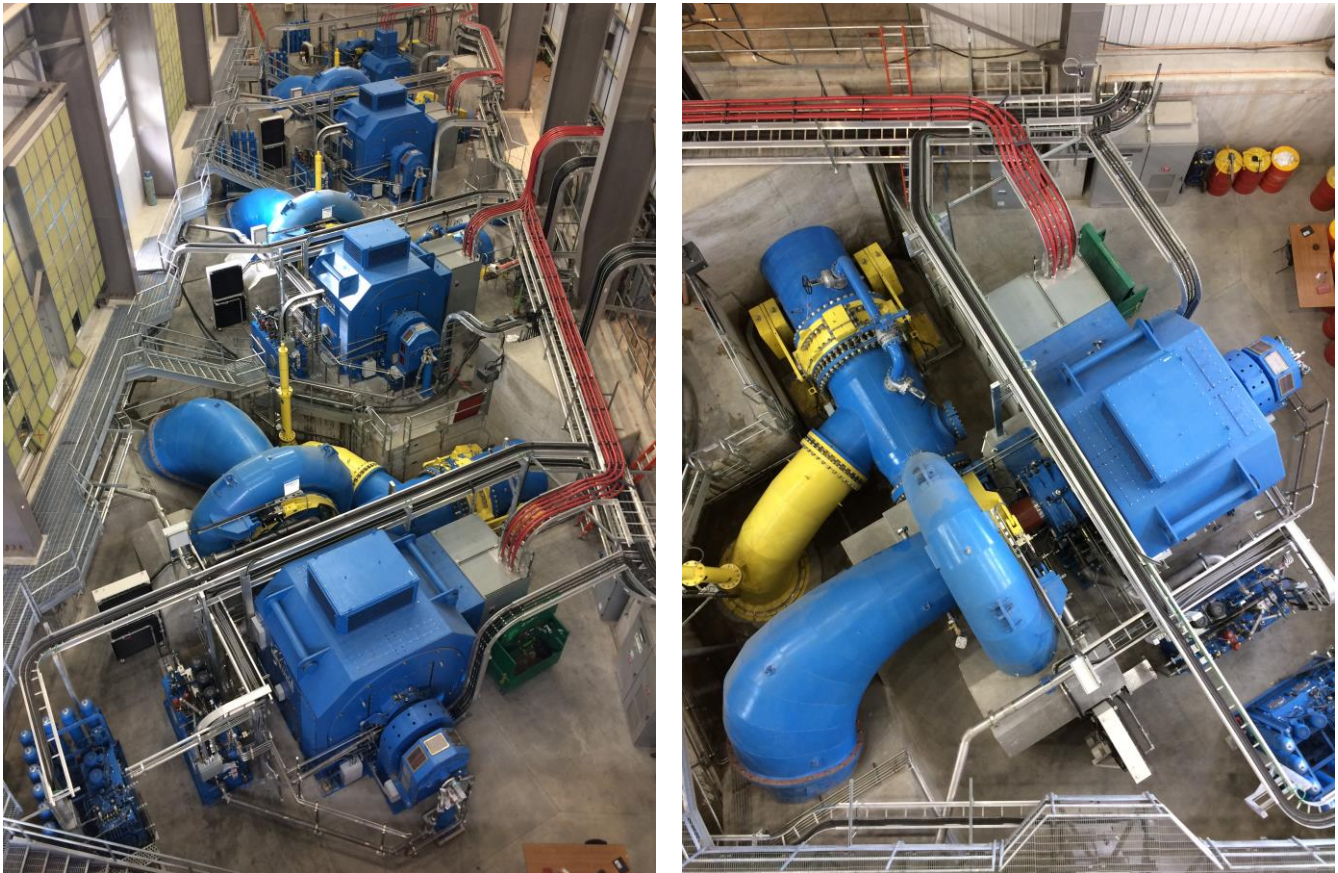
Appendix Figure: Photos of an example installation of similar horizontal Francis units
