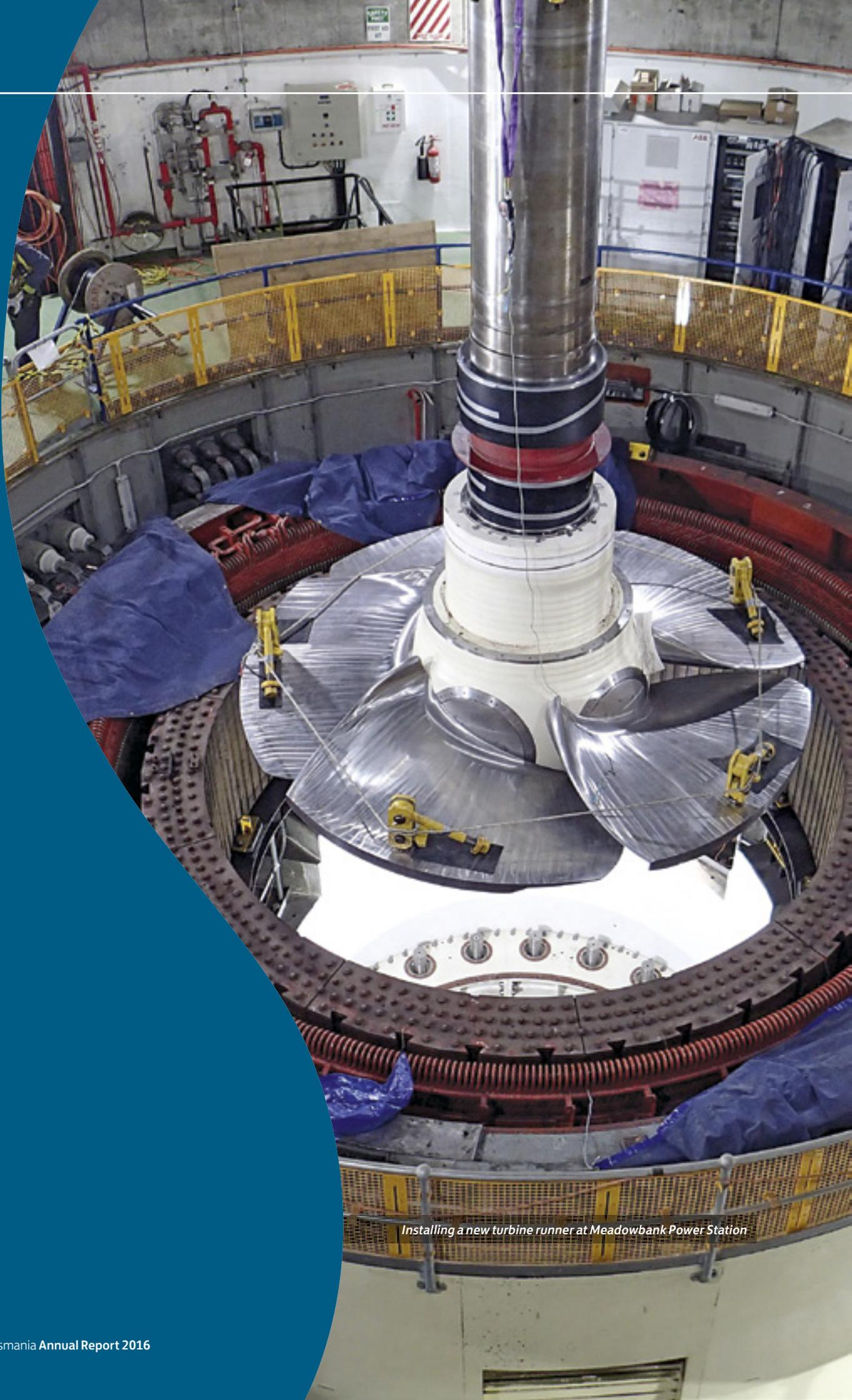
*Installing a new turbine runner at Meadowbank Power Station*
