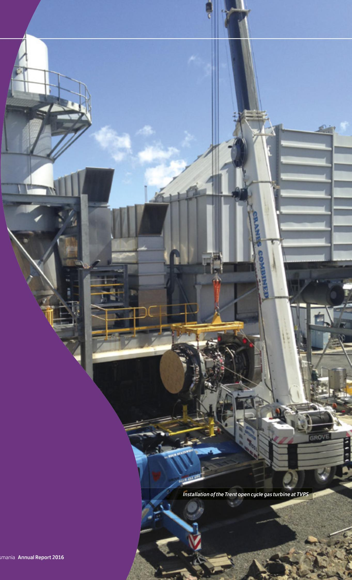
*Installation of the Trent open cycle gas turbine at TVPS*
