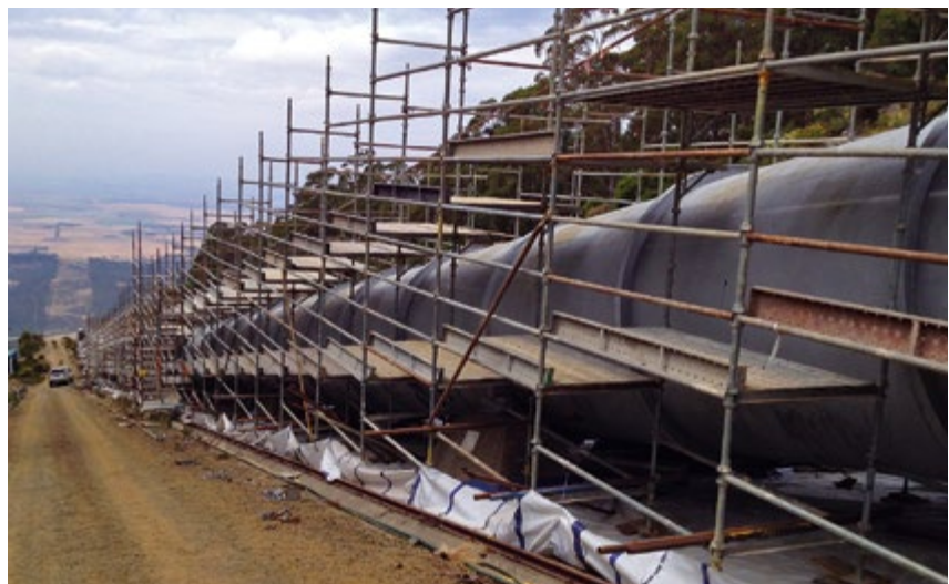
Painting the Poatina Penstock after 50 years' service; it is 1.5 km long, 2.9 m diameter
