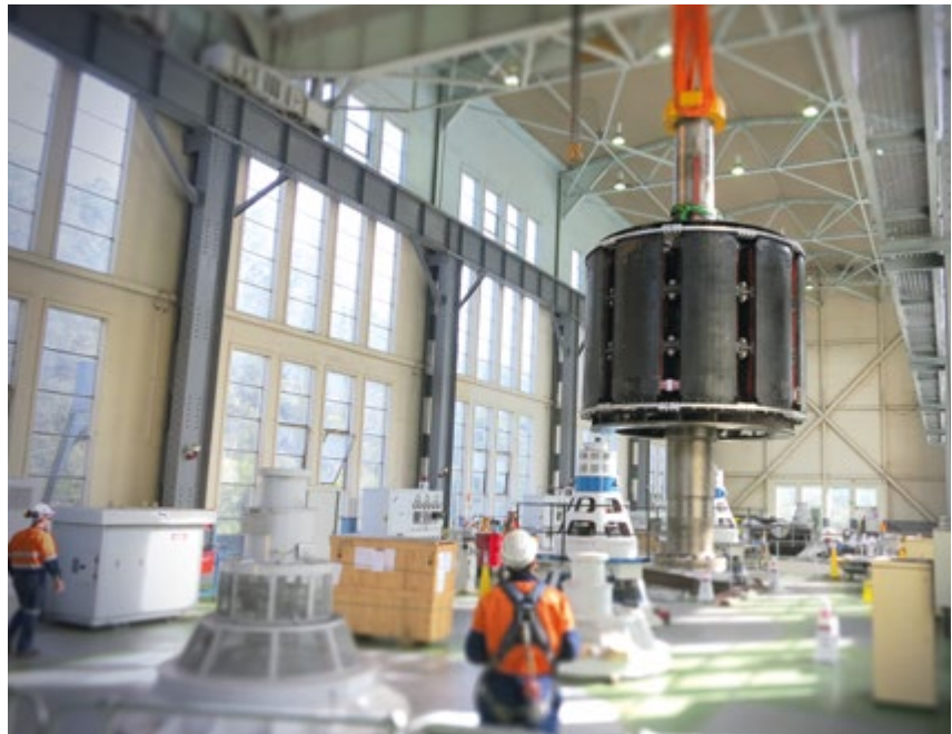
Tungatindah Power Station modernisation: lowering a rotor into place
