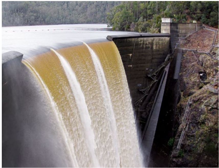
Spill at Devils Gate Dam
