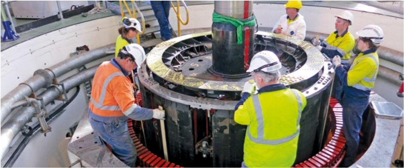
Tungatinah Power Station modernisation: employees and contractors installing a rotor
