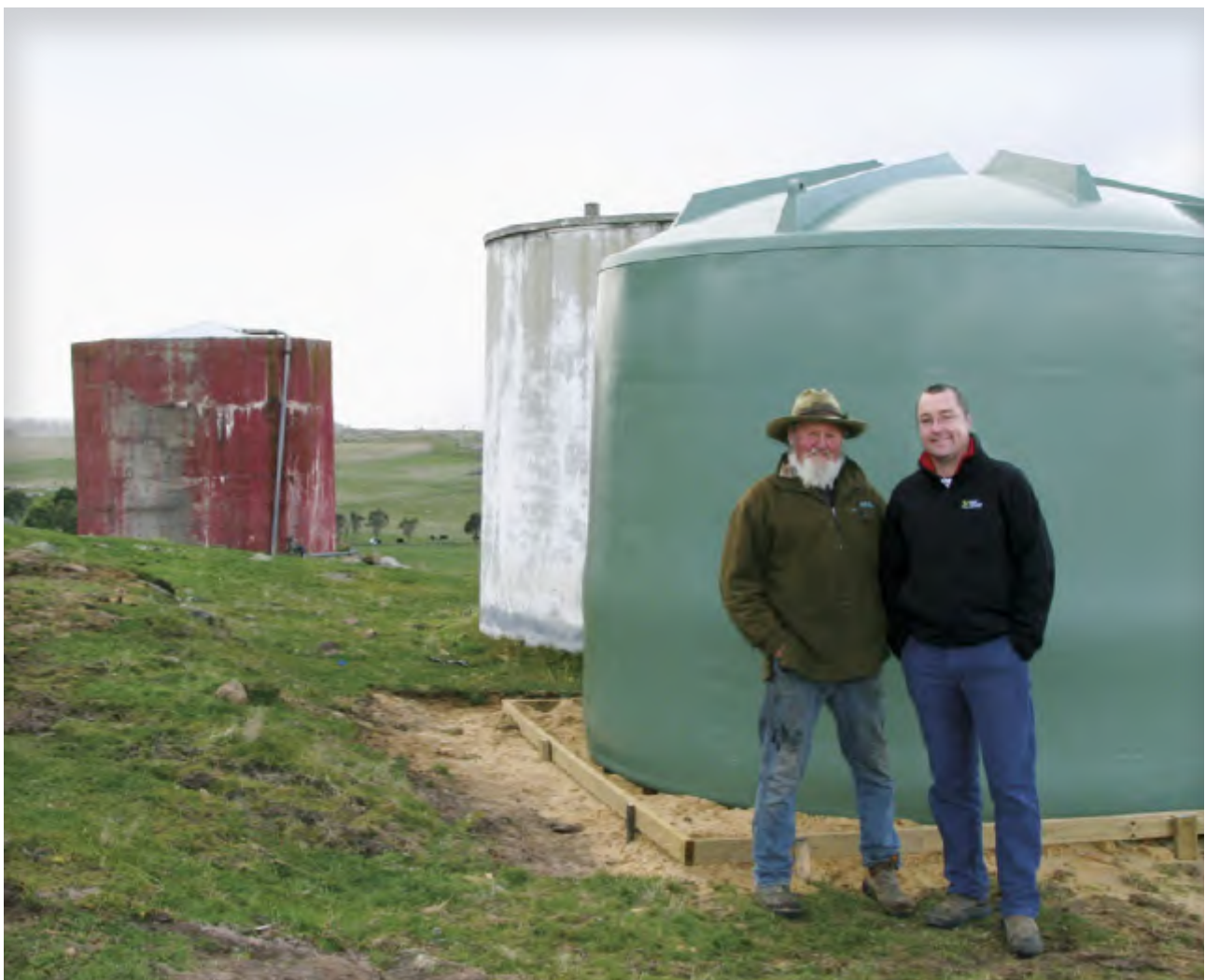
Hydro Tasmania's Andrew Jones, right, with Shannon River resident Rob Casey in front of one of the new water tanks
