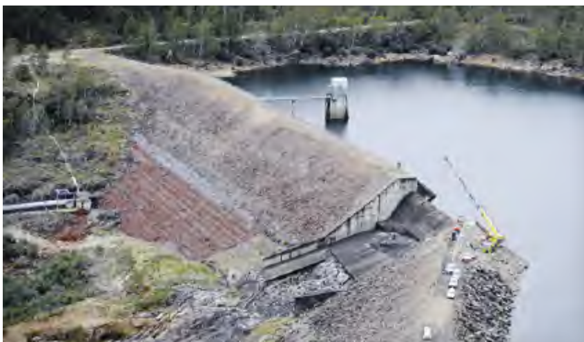
Rowallan Dam, where a major spillway upgrade will soon begin
