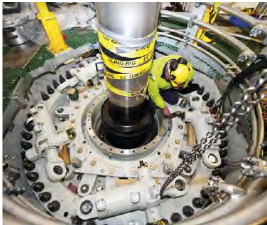
Refurbishment work at Tungatinah power station
