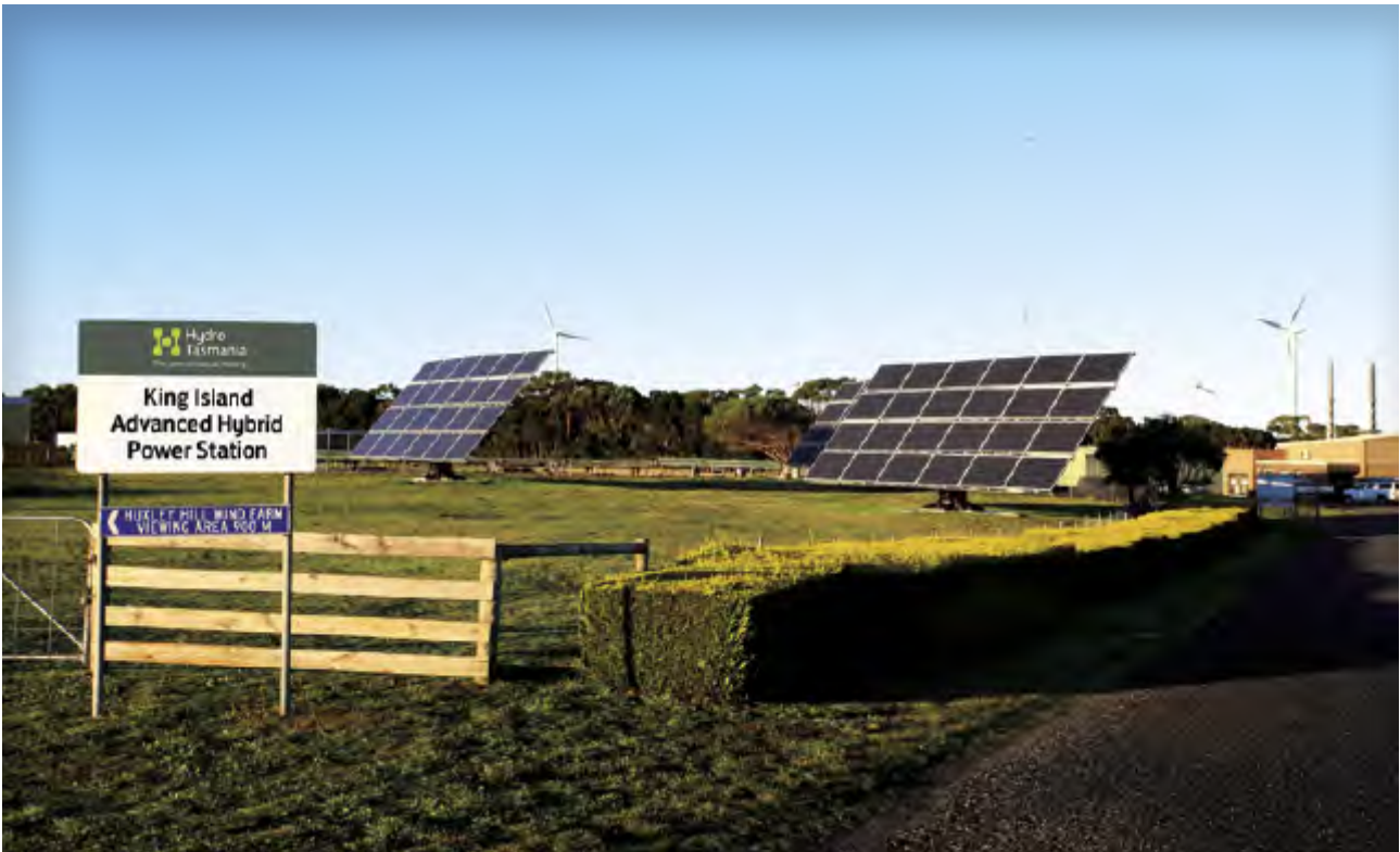
The King Island advanced hybrid power station uses a combination of renewable energy and diesel
