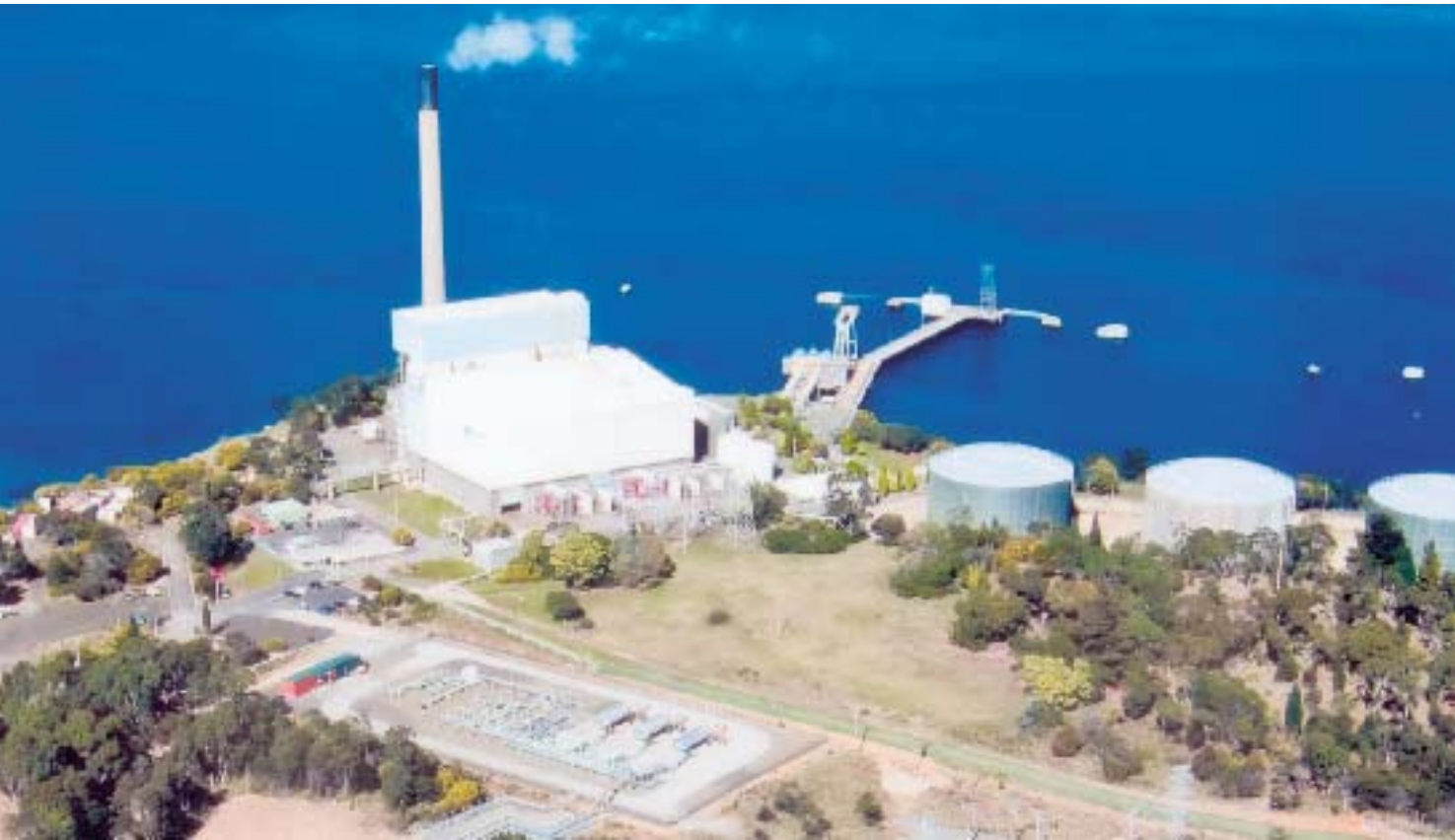
Bell Bay Power Station
