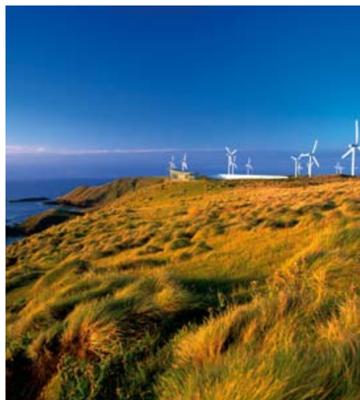
Woolnorth Wind Farm
