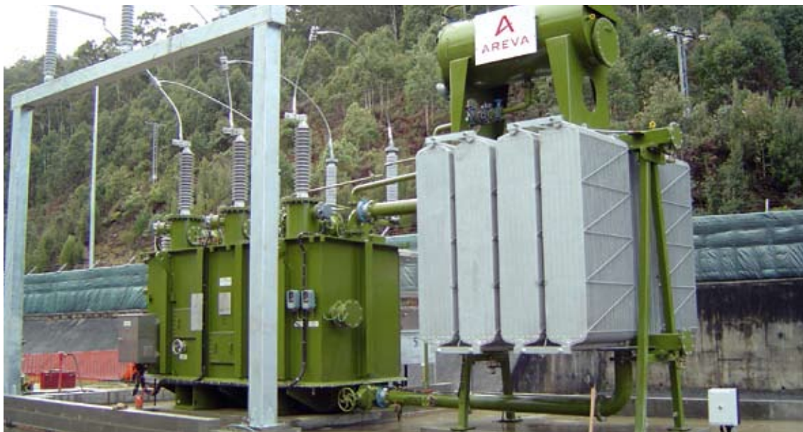
The successfully recommissioned Tungatinah No. 5 transformer
