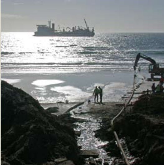
The Basslink cable comes ashore
