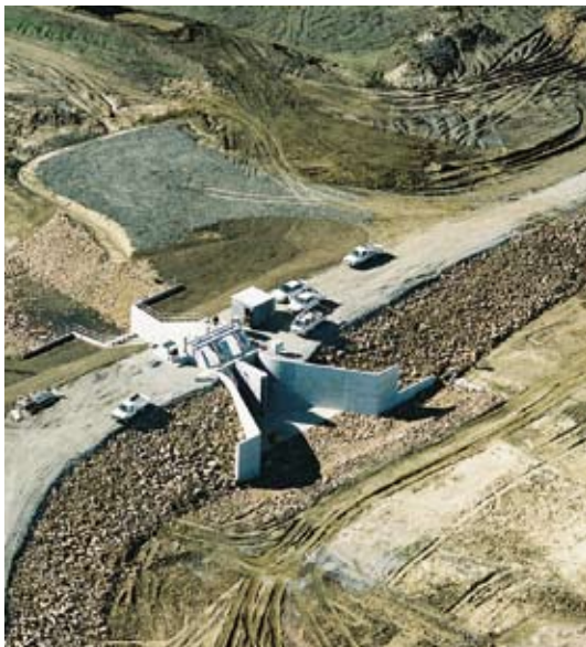
The Poatina re-regulation pond under construction
