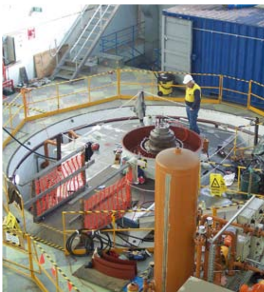
Safety in practice – Trevallyn Power Station upgrade project
