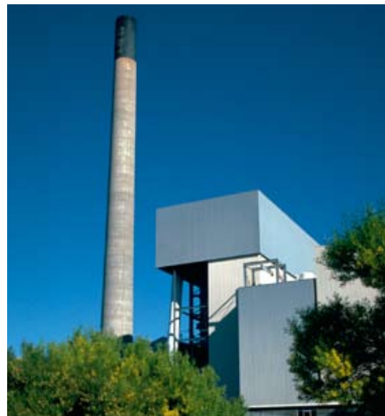
Bell Bay Power Station
