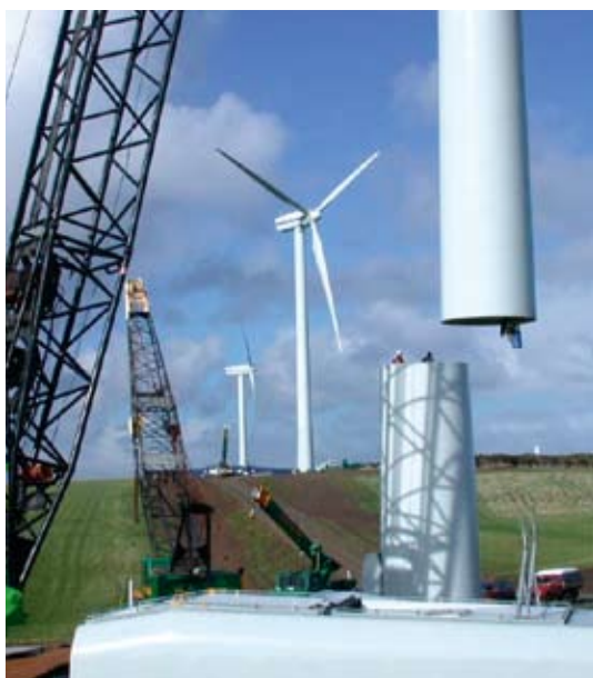
Work nears completion on Woolnorth Wind Farm Stage 2
