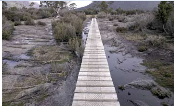
The boardwalk near the Narcissus River showing jute matting and slash laid previously by PWS to encourage vegetation regrowth
