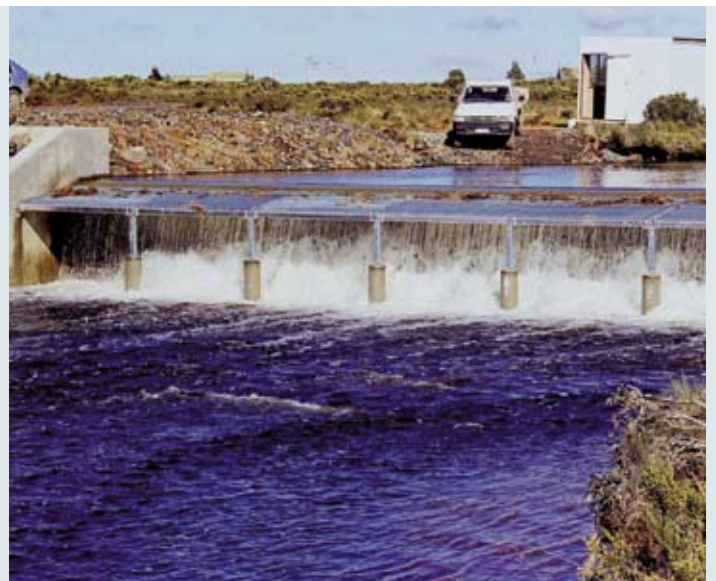
Natural or man-made barriers like this one in Liawenee Canal prevent the spread of redfin perch
