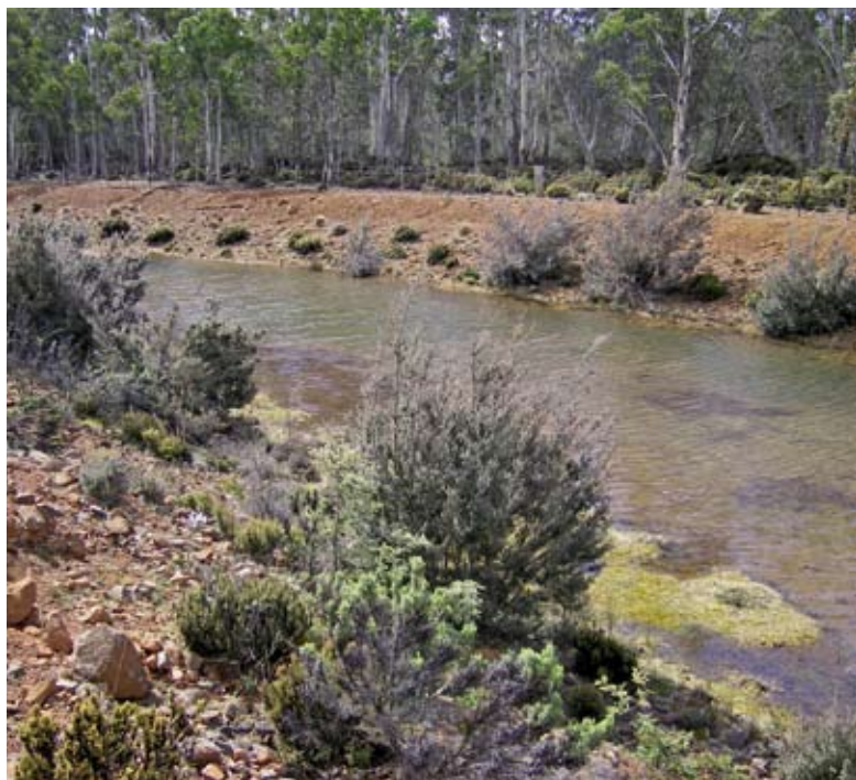
Waddamana Two Canal prior to installing the bunds (9 October 2006)
