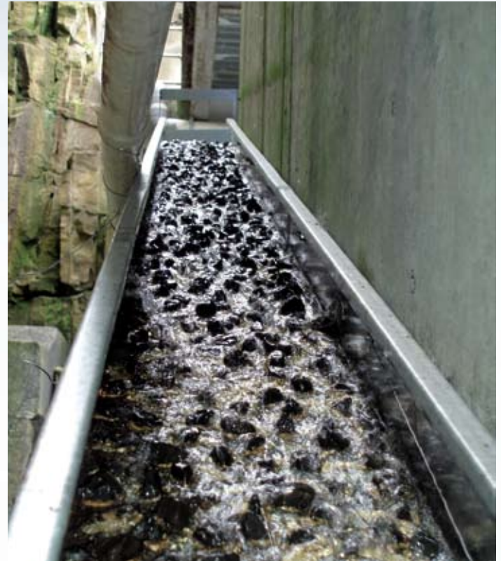
Access ramp to fish trap. The rock lining helps the elvers climb to the trap
