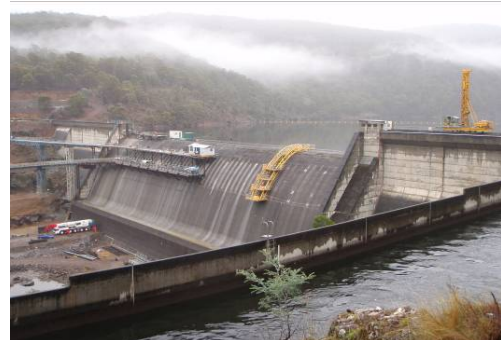
Work in progress at Catagunya Dam
