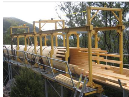
Woodstave pipeline under construction within mobile working platform
