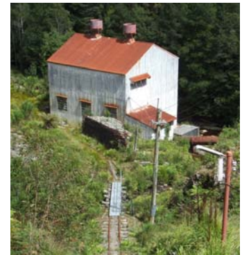
The lower Lake Margaret Power Station
