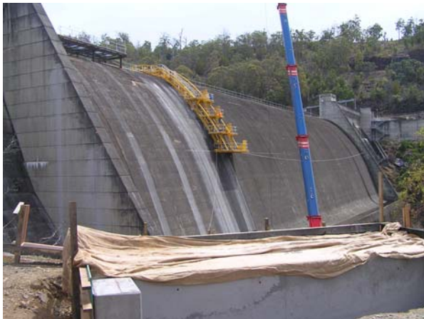
Catagunya Dam refurbishment in progress
