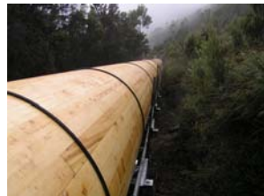
A section of the new pipeline constructed from Alaskan Yellow Cedar
