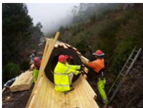
The new pipeline under construction at Lake Margaret
