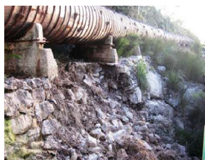
A preserved section of the 1938 woodstave pipeline at Lake Margaret
