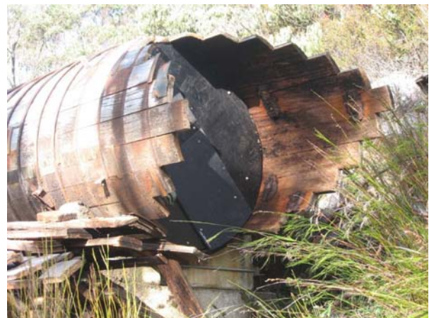
Lake Margaret woodstave pipeline preserved section 2007
